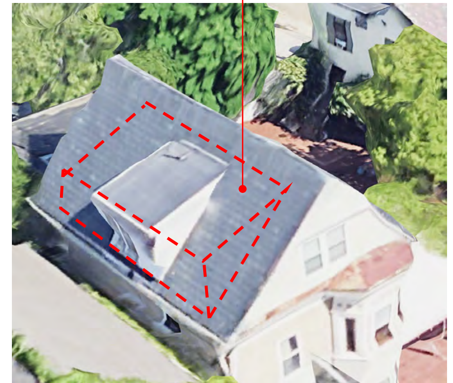
Aerial View / North Roof – Current 2023
