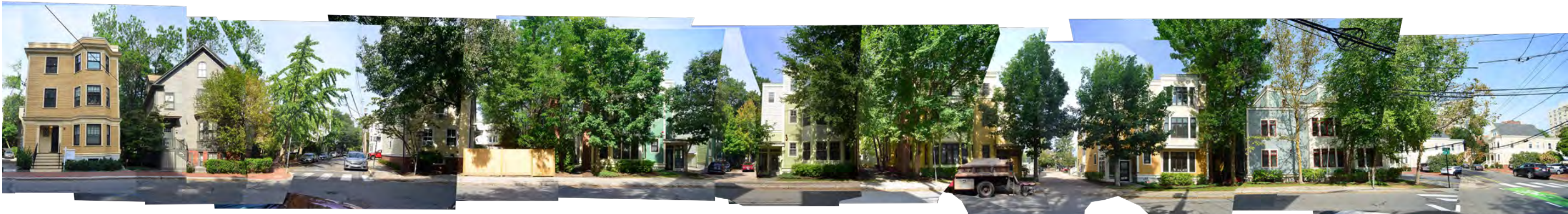
Grant Street – north side
