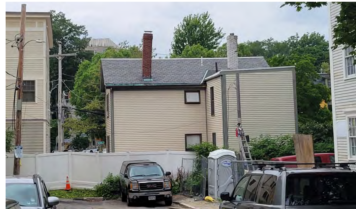
East Elevation (view from Green Street) – Current 2023
