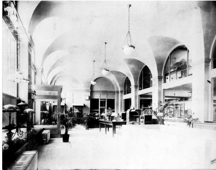
727 Massachusetts Avenue, Cambridge Gas-Light building. Interior view, 1914.
