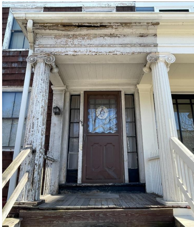
196 Prospect Street, entry detail.
