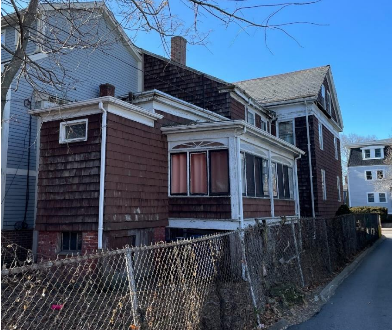
View of 1899 one-story Louis (Lewis) F. Baldwin addition and bathroom and enclosed porch added by a later owner, facing Prospect Street.
