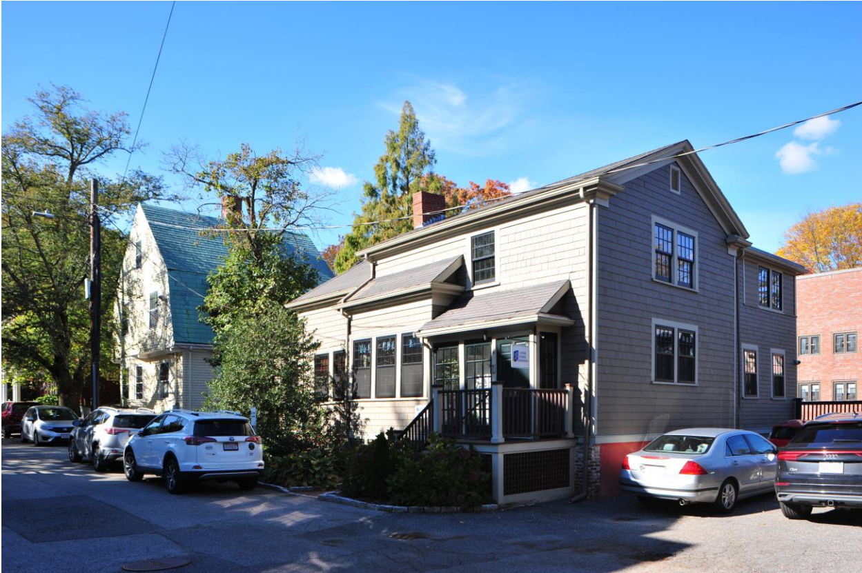
South and east elevations of 6 Buckingham Pl. Two-story addition at right. CHC staff photo, Nov. 2021.
