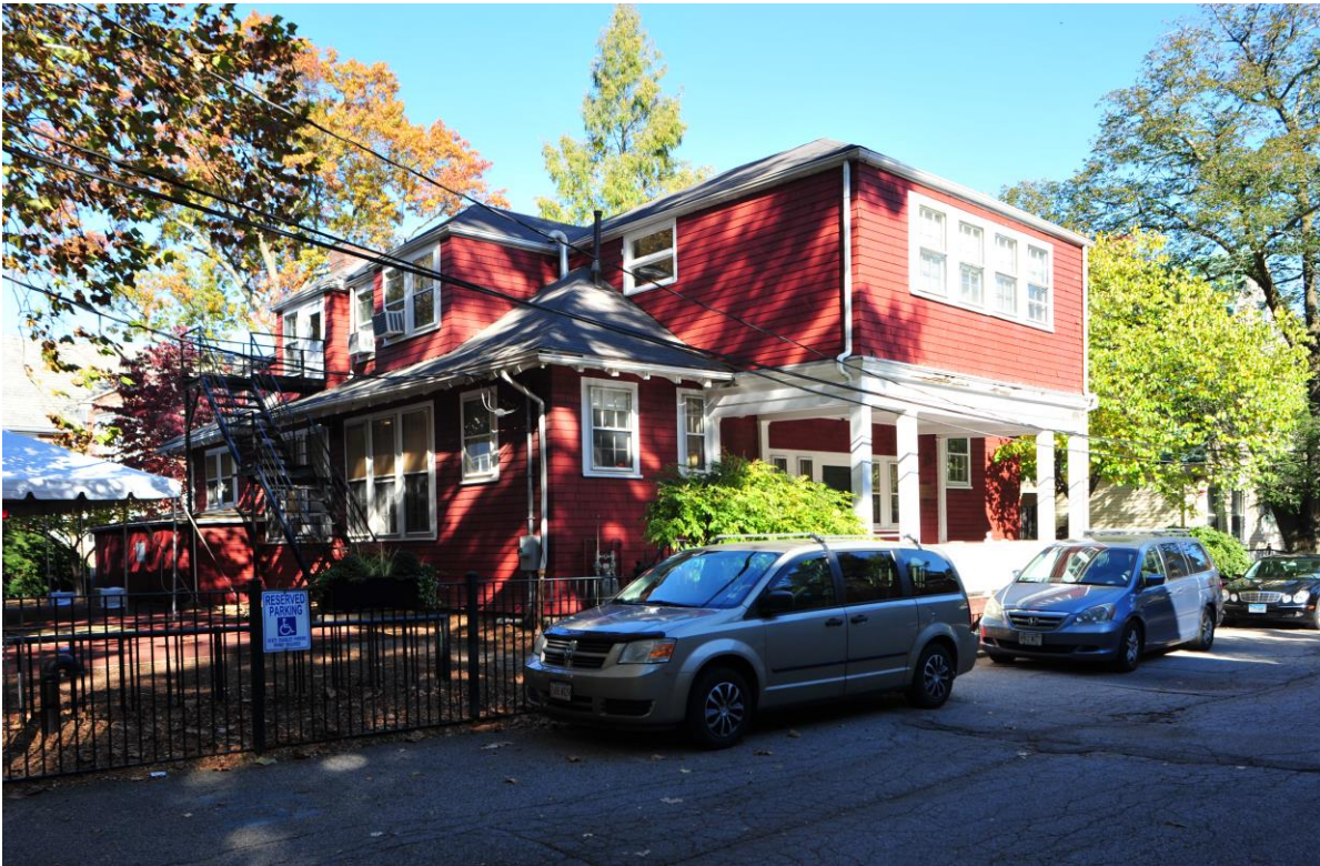
West and south elevations of the Markham building at 10 Buckingham St. CHC staff photo, Nov. 2021.
