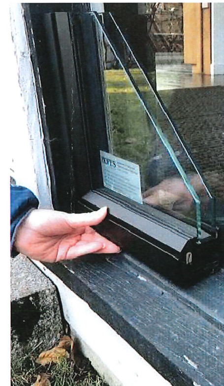
Existing Fixed Window with Proposed Hope Landmark Profile
