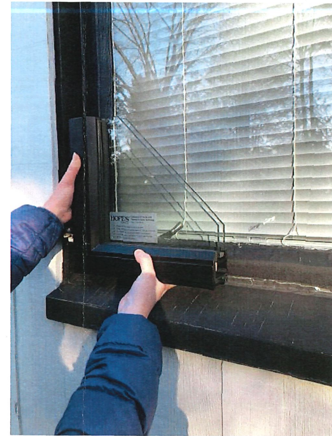
Existing Operable Window with Proposed Hope Landmark Profile
