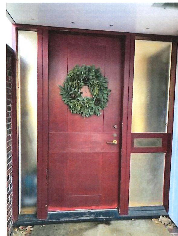
Existing Condition At Front Door
