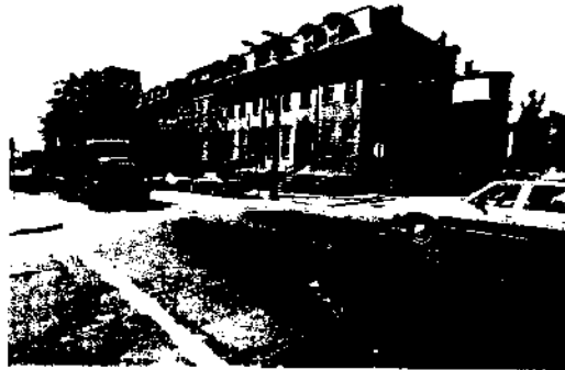
27. Third Street. Photograph shows heavy truck through-traffic.
