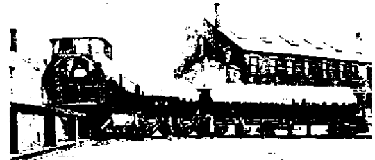
14. The Meigs Elevated Railway. This railway was an experimental forerunner of rapid transit development in America. This photograph of 1887 shows the cylindrically-designed steam locomotive, tender, and car posed on the monorail structure in East Cambridge. The railway performed very well under extensive testing and was open for public demonstration in 1888. Unfortunately, it was felt to be a little ahead of its time and never became a part of Boston's rapid transit system.
