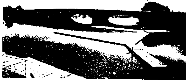
38. Eliot Bridge, Charles River The new Lechmere Canal Bridge will be designed to be a graceful addition to the Charles River Basin.
