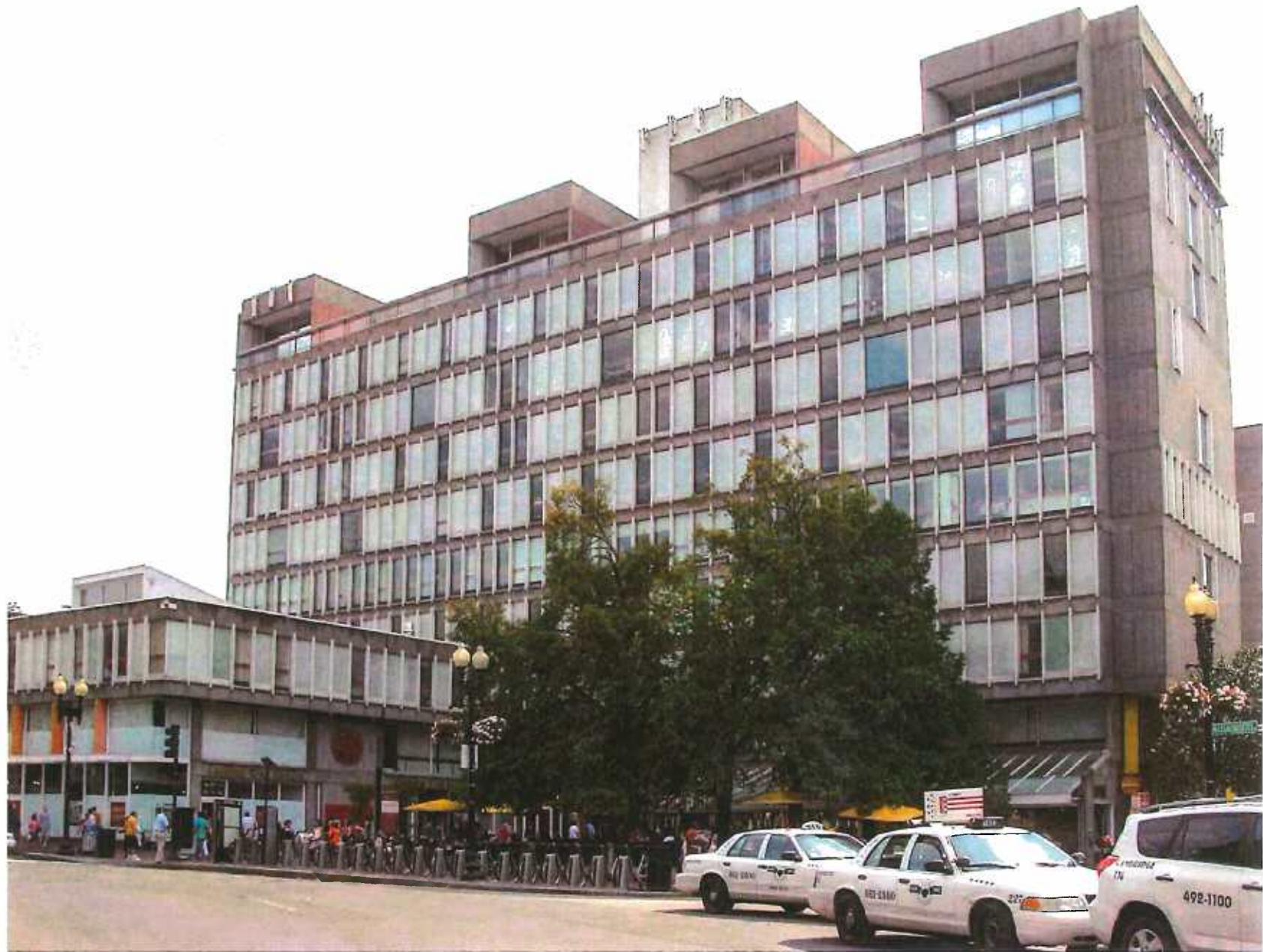
1350 Mass Ave Smith Campus Center – Currently Under Renovation (Pavement Coffee House)
