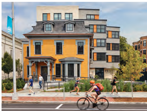
The completion of Frost Terrace in FY22 brought 40 new affordable housing units to Porter Square. Photo: Robert Benson Photography
