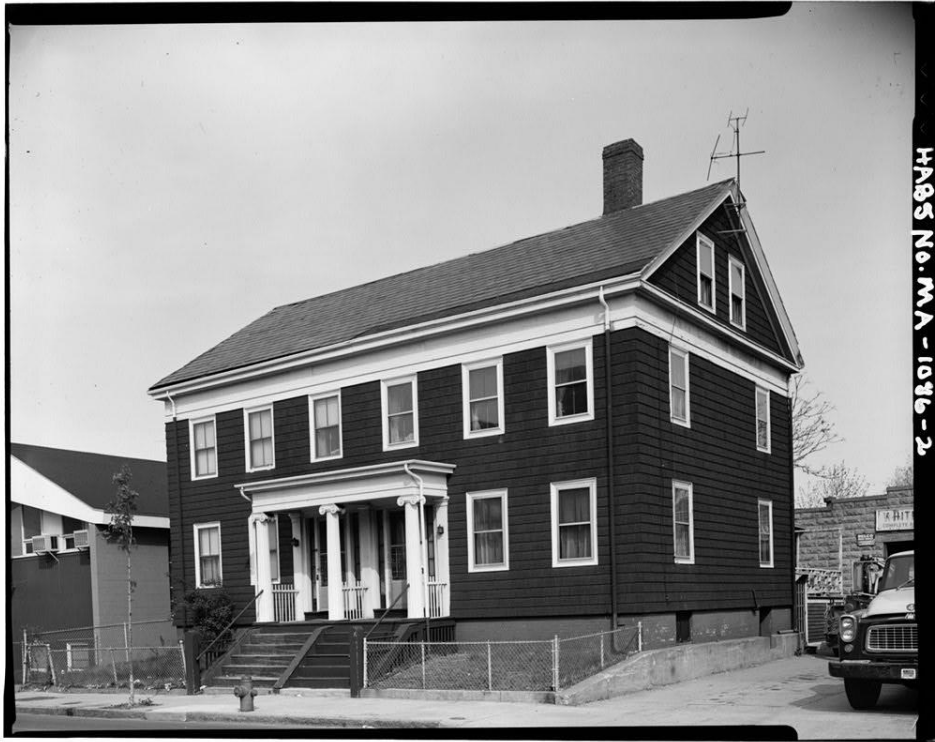
194-196 Prospect Street, c.1970. Historic American Buildings Survey photograph.
