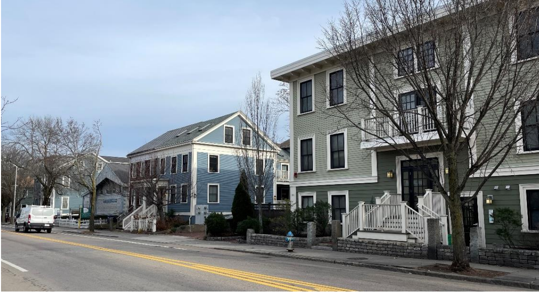
Looking north on Prospect Street, 194-196 Prospect St at center-left. CHC staff photo, 2022.
