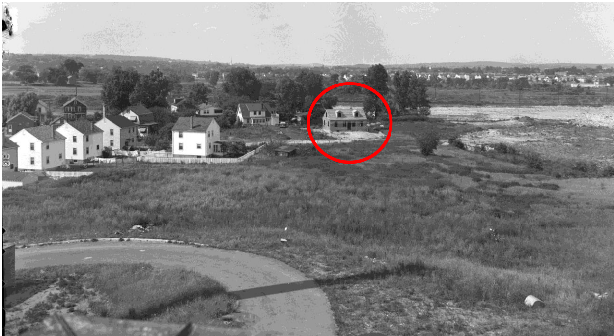
21 Loomis Street under construction, as seen from the roof of the Cambridge Sanatorium, 1949
