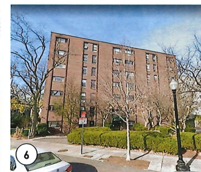
6 101 WESTERN AVENUE 7 STORIES RESIDENTIAL BUILDING
