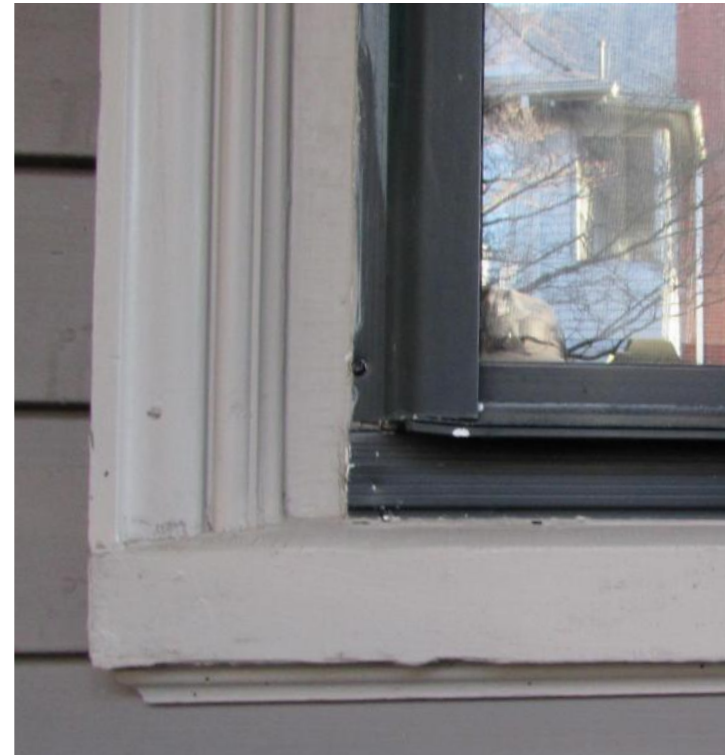
IMAGE OF EXISTING WILL SILL, APRON AND CASING
