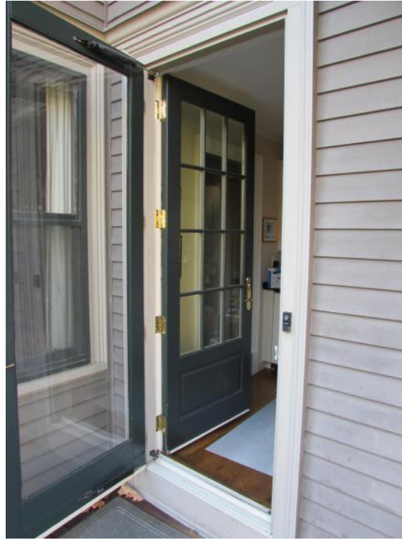
EXISTING DOOR #2 TO BE REMOVED
