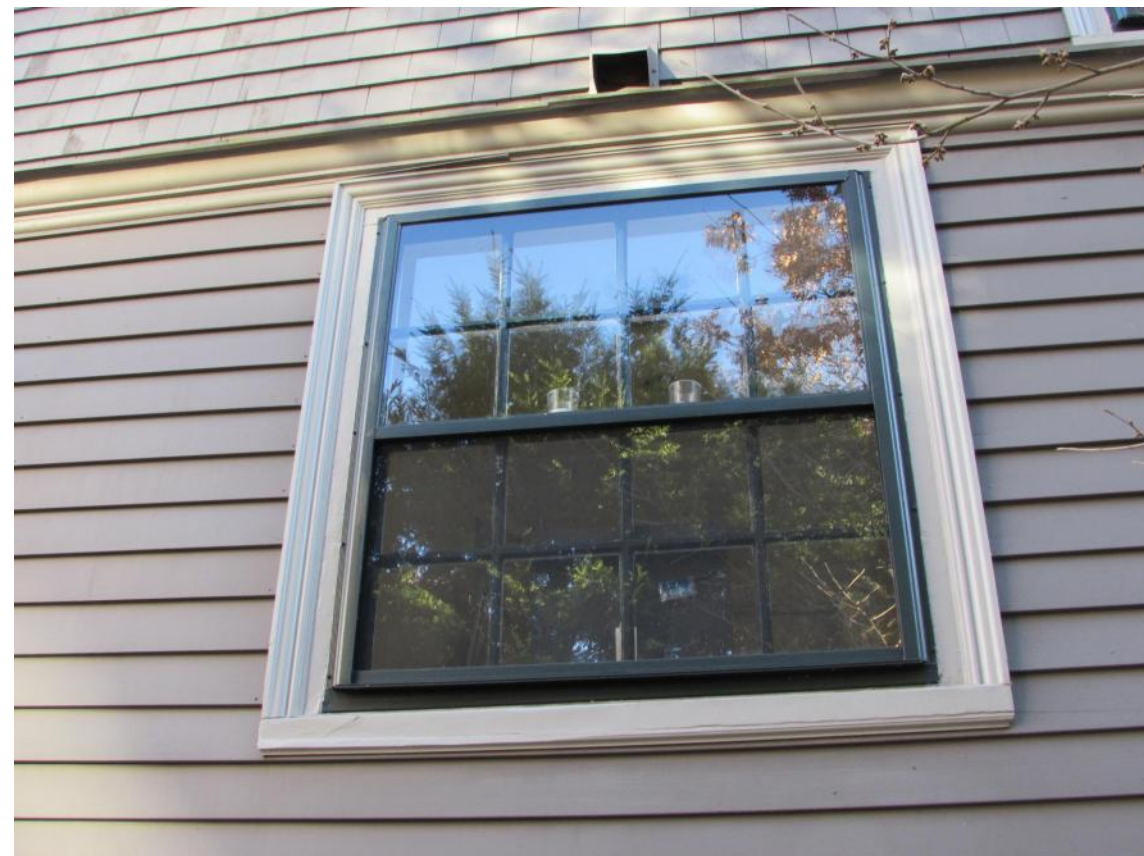
EXISTING WINDOW #6 TO BE STORED FOR POSSIBLE FUTURE REUSE
