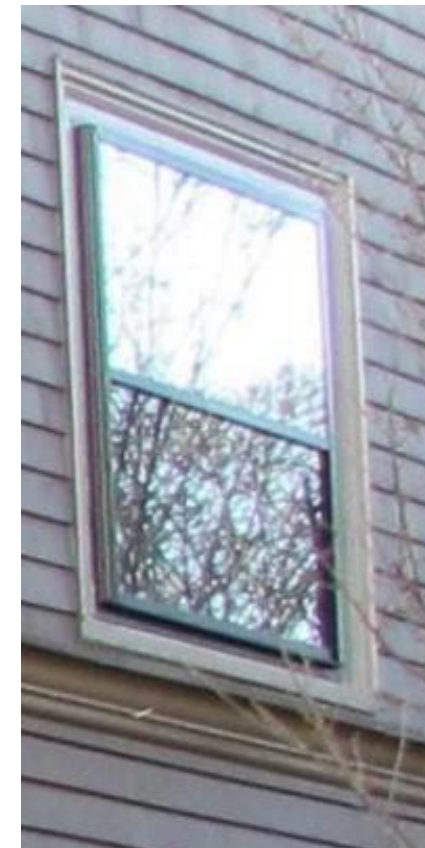
EXISTING WINDOW #7 TO BE STORED FOR POSSIBLE FUTURE REUSE
