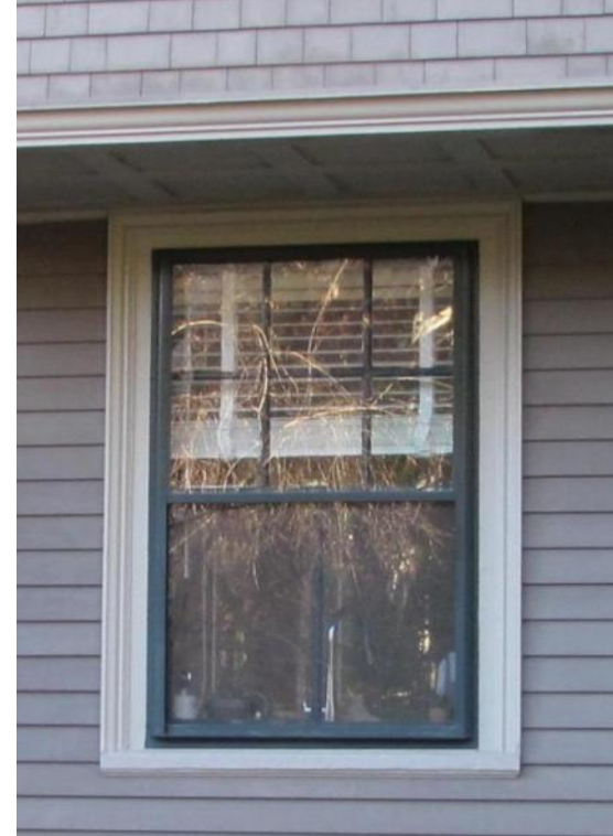
EXISTING WINDOW #3 TO BE REUSED
