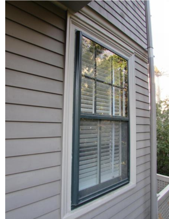
EXISTING WINDOW #4 TO BE REUSED
