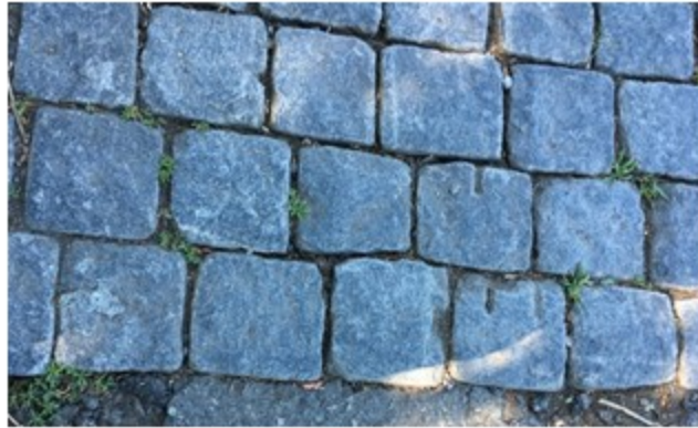
Existing Pavers at Longfellow Park
