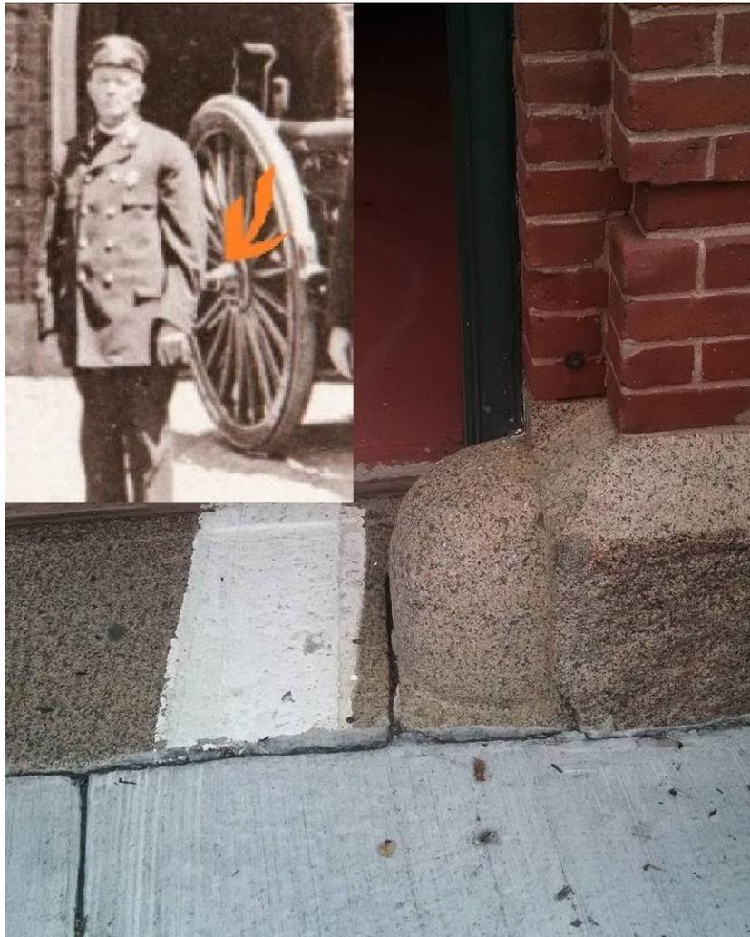
The exact name for them is a bollard, but quite simply they were installed just to protect the apparatus (which at the time were steam engines) from bumping into the very solid walls of the stations. The steamers and carriages had long wheel hubs (*see orange arrow in insert photo*) approximately 8" long. If the wooden wheel were allowed to brush against the brick wall while entering or exiting, it could do damage to the wheel rendering the apparatus unable to respond if the hub were damaged.
