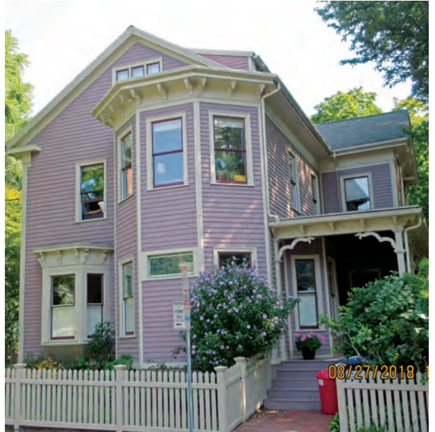
A 2018 view of 32 Avon Hill Street, the house Huntington built for his orphanage (later called the Avon Home). City of Cambridge Property Database
