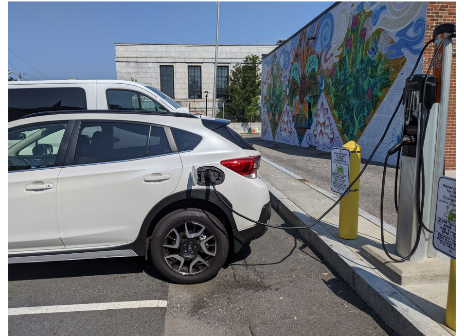
Lot 8 EV Charger
