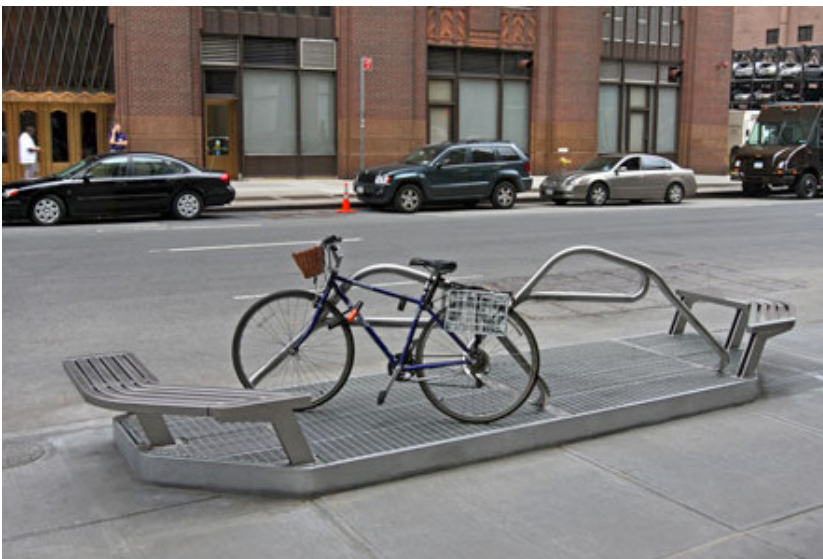
Figure 30. “Raised-grate street sculptures to prevent subway flooding. Stormwater improvements have been made at chronic flood locations by integrating raised-grate street sculptures to prevent subway flooding within the MTA NYCT service area and also serve as street furniture and/or bike racks.” Metropolitan Transportation Authority, New York City. 65
