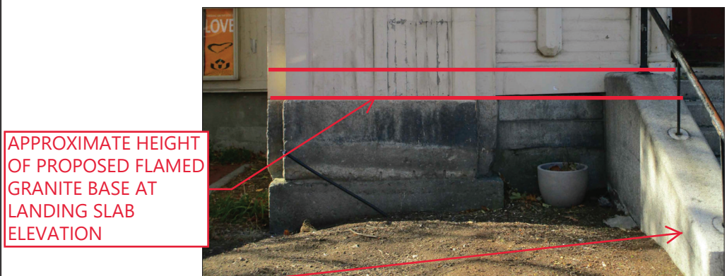
EXISTING EXPOSED FOUNDATION WALLS, TYP
