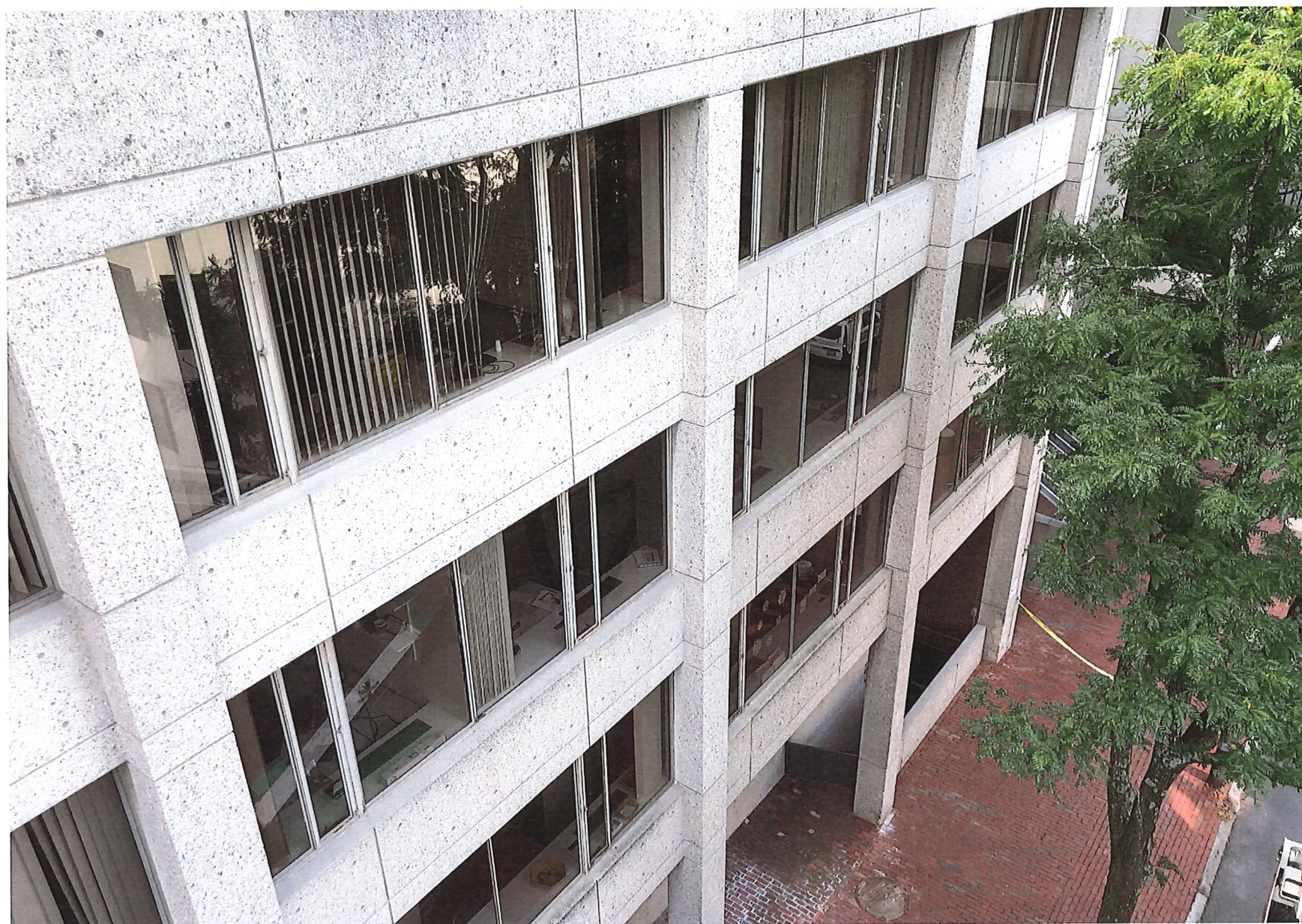
8 Story St (North) Photo from aerial lift
