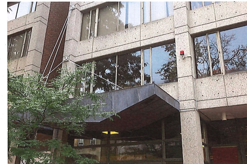
North facade - entry with overhang
