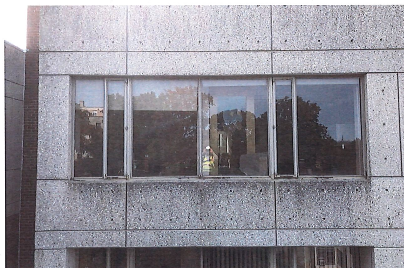
Window unit - 5th floor, North facade
