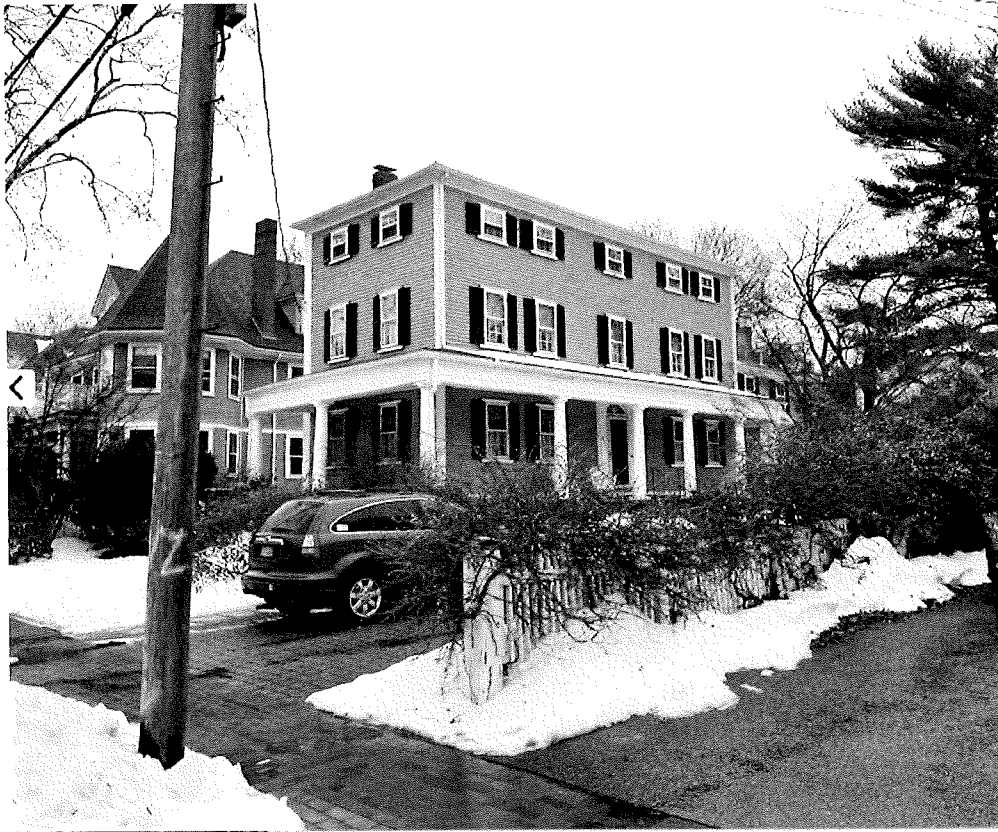
Panel C1: 10 Frost Street, south elevation from the street
