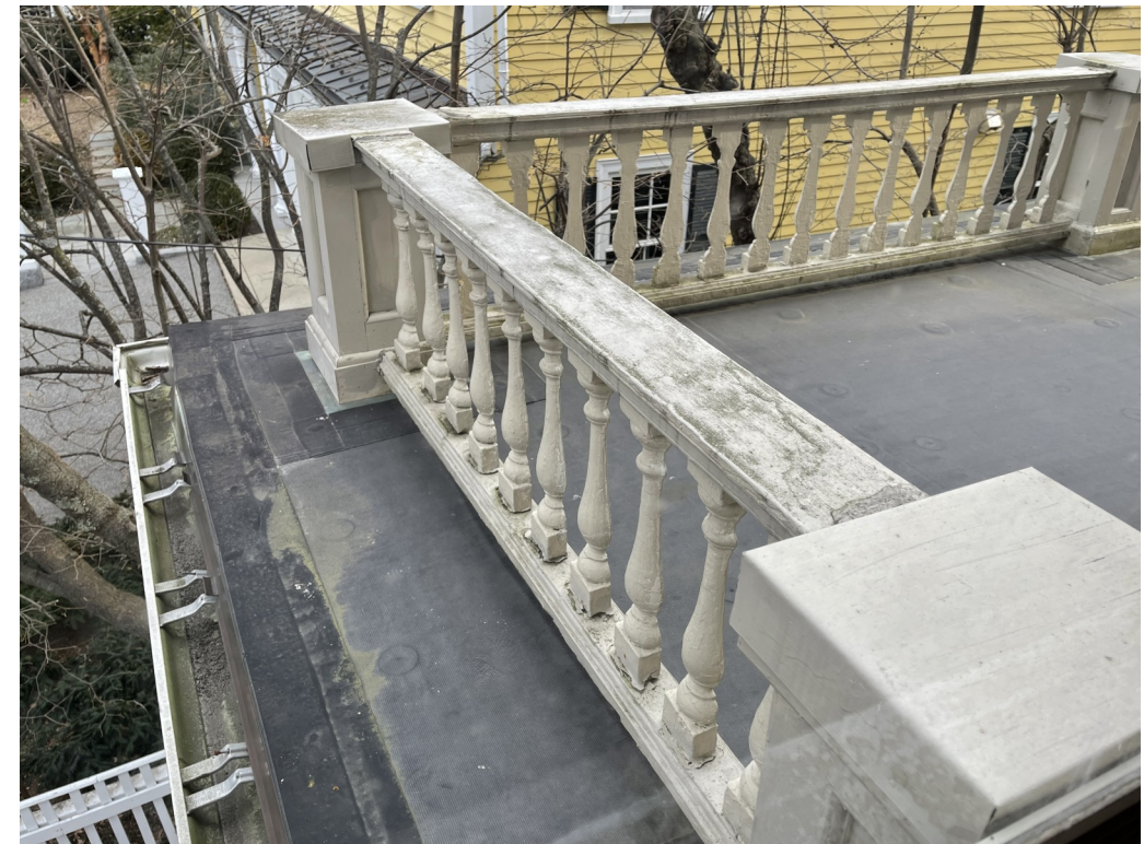
RAILING ON RIGHT OF HOUSE
