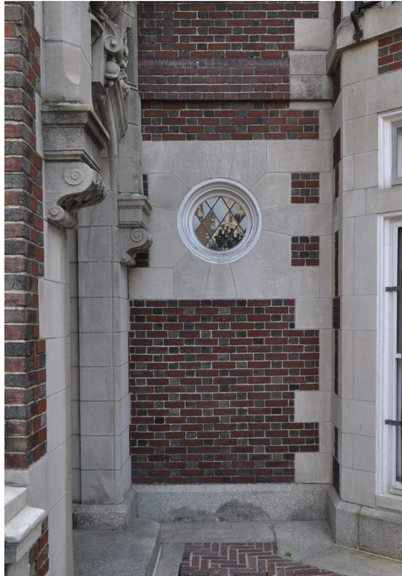
1. PHOTO - EXISTING CONDITIONS
