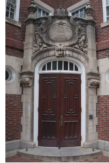
EXISTING A-ENTRY DOOR
