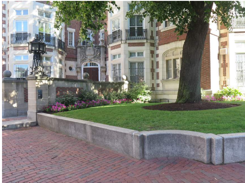
PHOTO - EXISTING CONDITIONS
