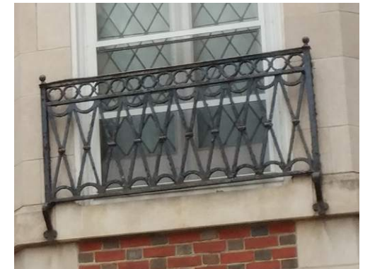
ADJACENT ORIGINAL 1902 METALWORK
