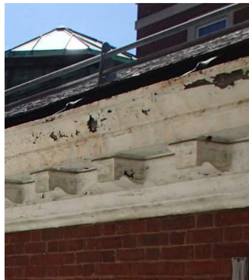
DINING HALL, PAINTED COPPER CORNICE WITH INTEGRATED GUTTER TO BE RESTORED
