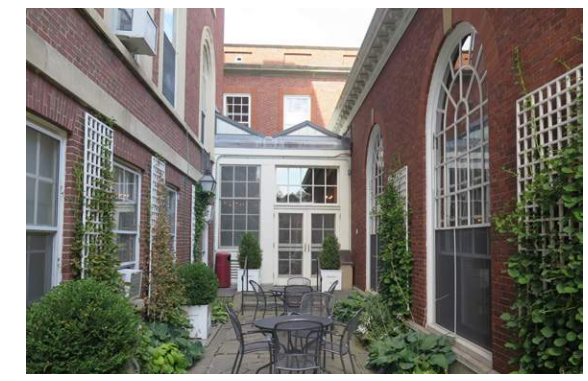
EXISTING CONDITIONS - PHOTOS
