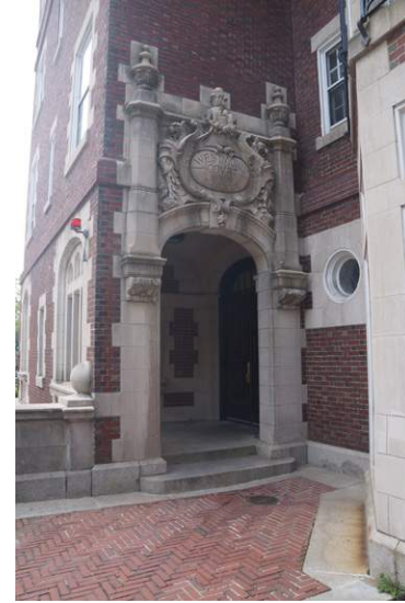
EXISTING B-ENTRY LOGGIA
