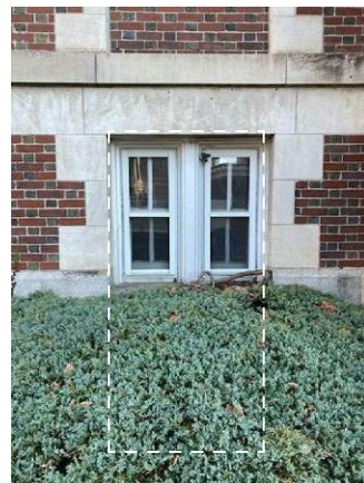
EXG CONDITION AT E.WG00C
