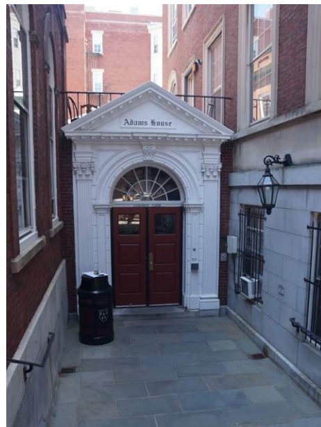
EXISTING ENTRY PHOTO
