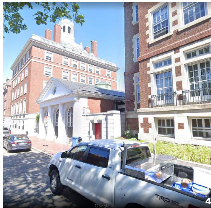
SOUTH FACADES OF 3 BUILDINGS FROM BOW ST.
