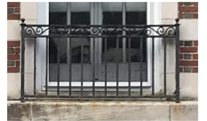
ADJACENT ORIGINAL 1898 METALWORK
