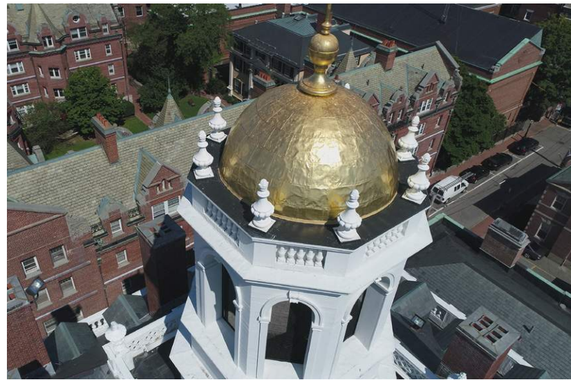
GOLD DOME TO UNDERGO MINOR REPAIR AND RESTORATION
