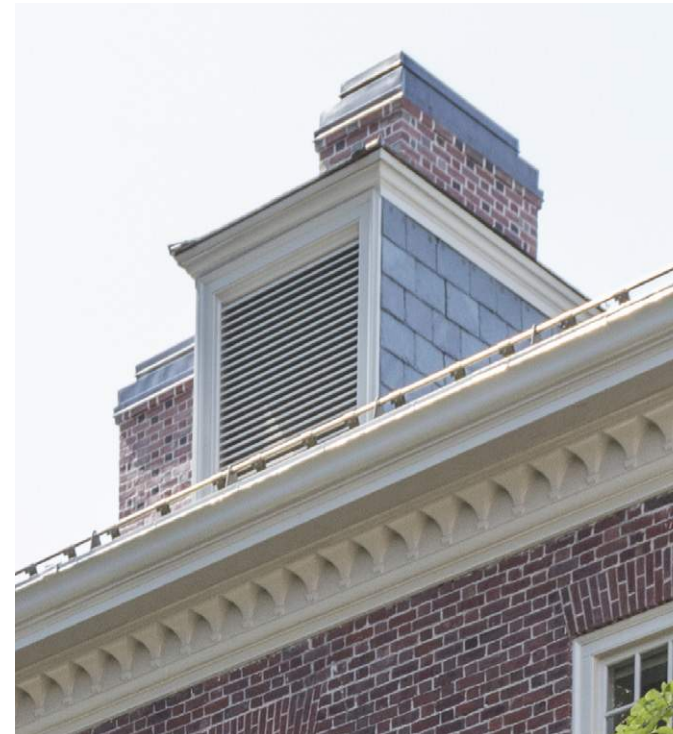
HISTORIC DORMERS AT WINTHROP HOUSE (SOME BECAME LOUVERED IN RENEWAL)
