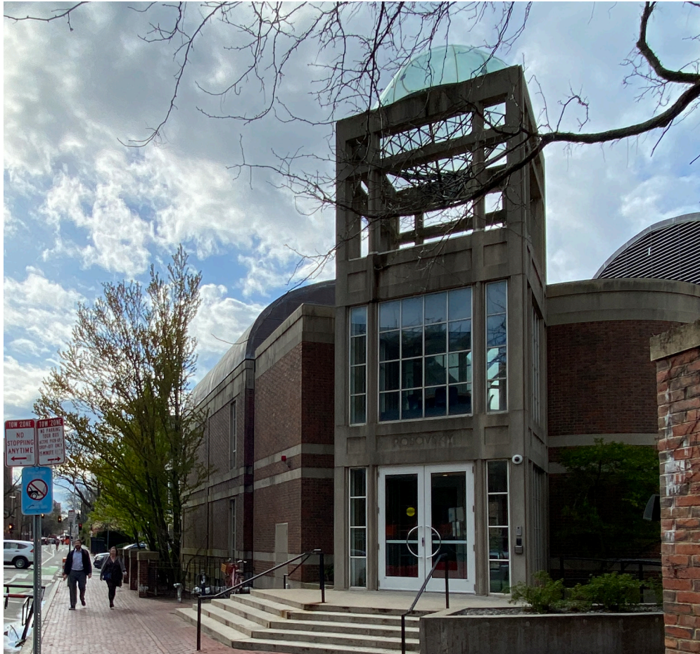
NORTH WEST ENTRY CORNER FROM MOUNT AUBURN STREET - EXISTING
