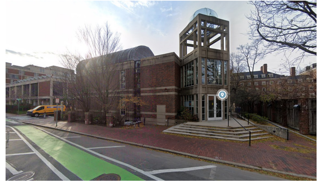
NORTH WEST CORNER FROM MOUNT AUBURN STREET
