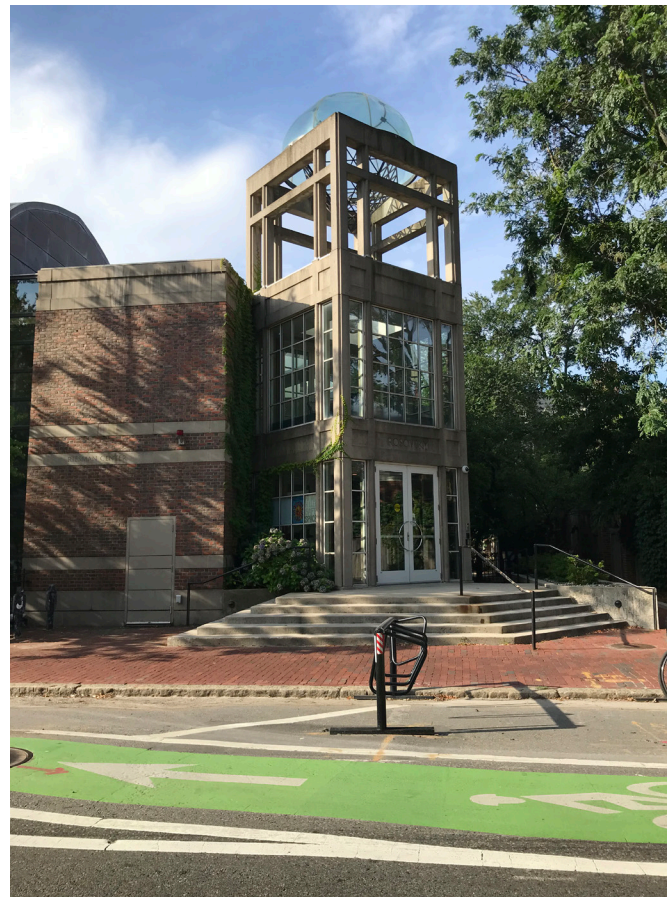
3. EXISTING ENTRY VIEW AT MT AUBURN STREET (MECH EQUIPMENT MAY BE MINIMALLY VISIBLE)
