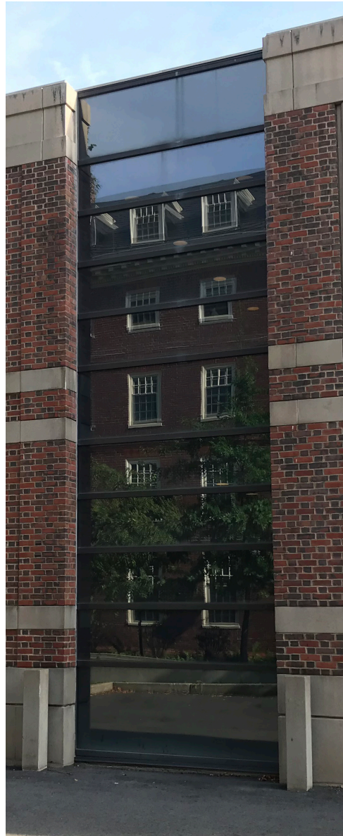
TYPICAL THROUGHOUT BUILDING
