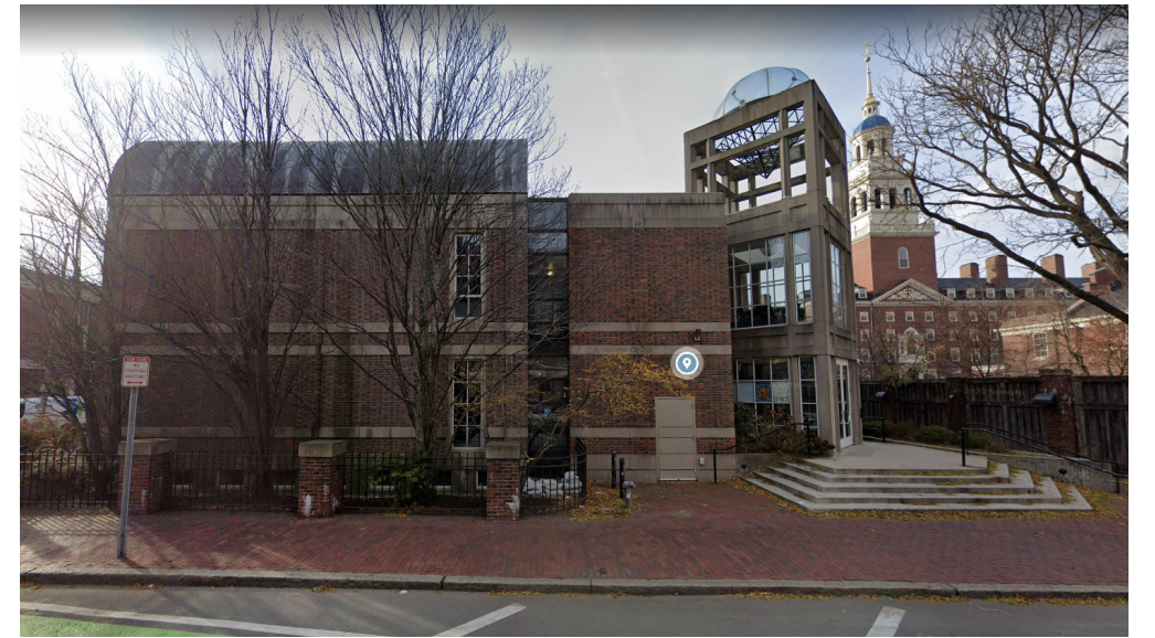
NORTH FACADE FROM MOUNT AUBURN STREET
