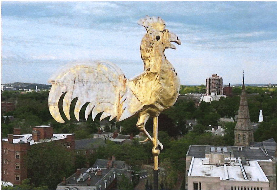
Drone photo taken of cockerel in place on tower– June 2023. Substantial damage to the surface finish was noticed.
