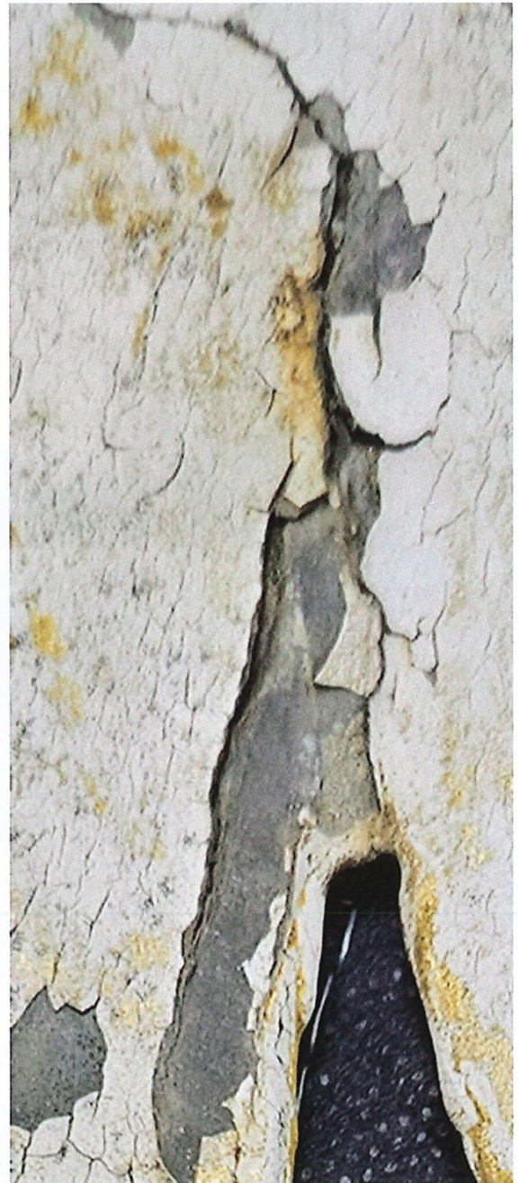
Crack between upper and lower feathers, worn side.
