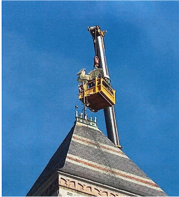
Steeple jacks removing cockerel weathervane from tower – November 2023
