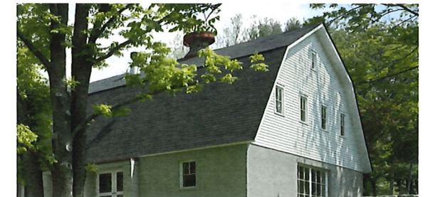
BARN / CARRIAGE HOUSE VERNACULAR
