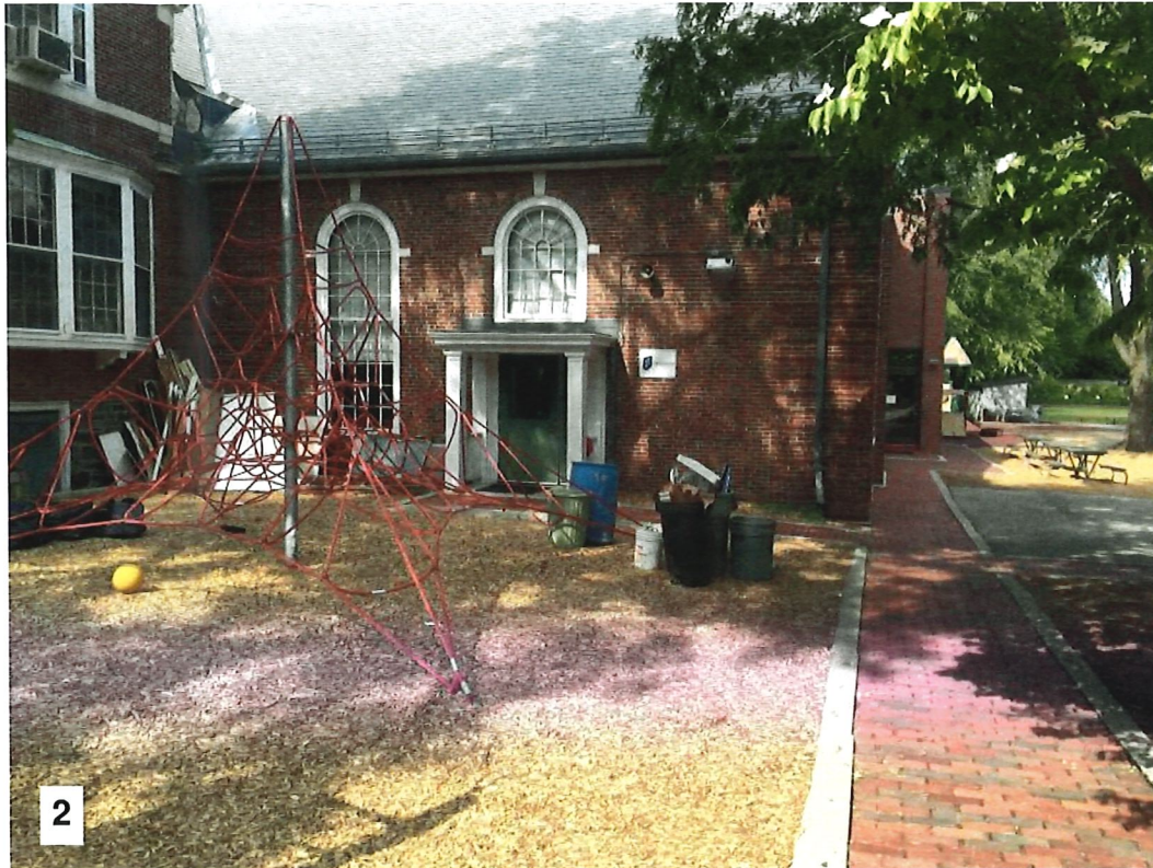
Brick Building at 16 Buckingham Street
