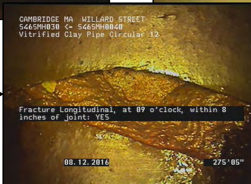
Example of infiltration (at joint)
