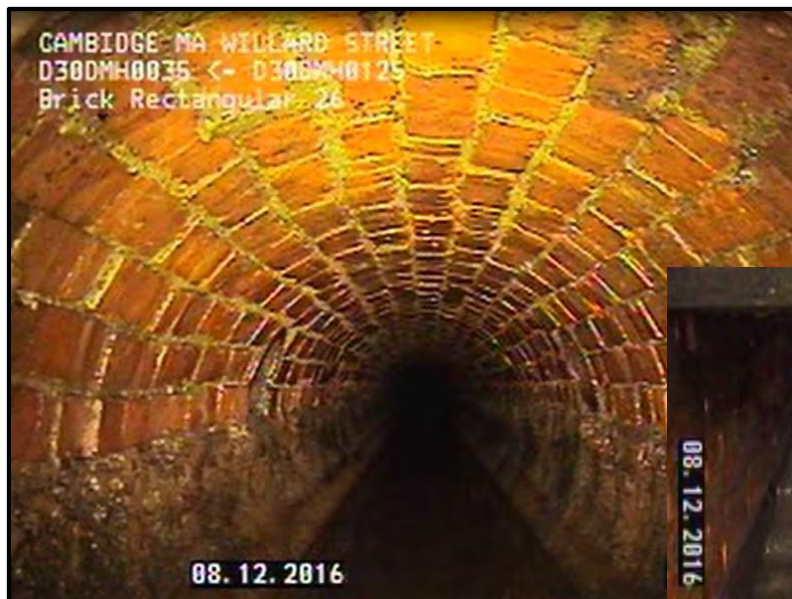
24"x 26" Brick sewer ↗
