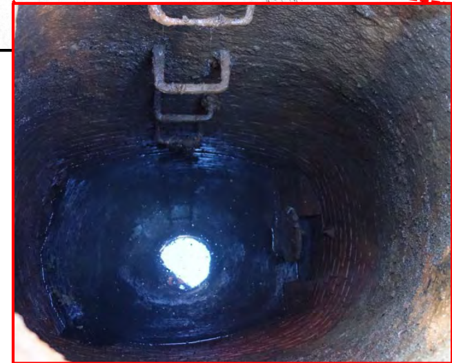
Access 032 Manhole at Regulator Structure (Sump)
