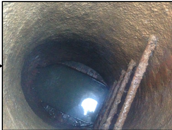
Regulator Structure Storm and Sewer Connections
