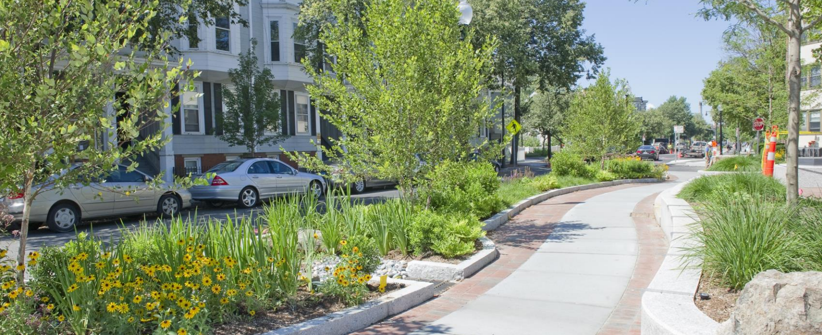
Rain garden installed at Western Avenue and Pleasant Street
