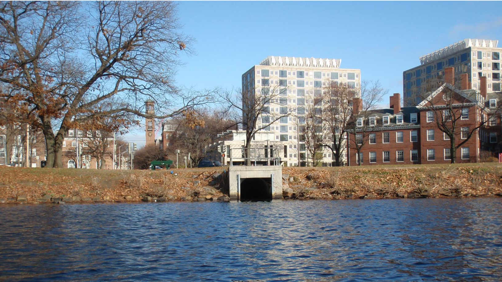
MS4 Outfall at Dewolfe Street
