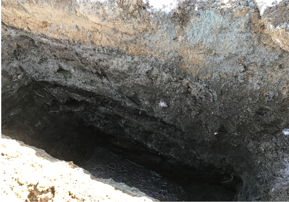
-Exposed north sidewall with groundwater at approximately 11' bgs
