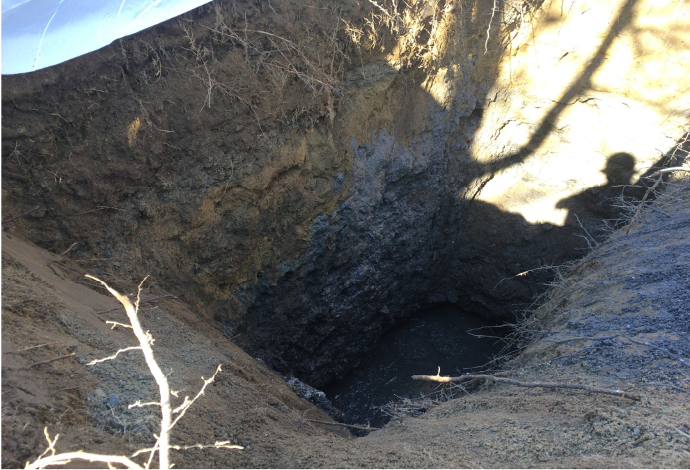
-Exposed west sidewall with groundwater at approximately 12.5' bgs
