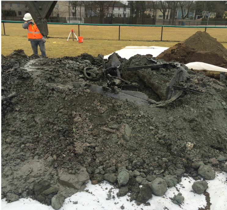
-Stockpile of waste fill material showing metal car frame removed at approximately 11' bgs.
