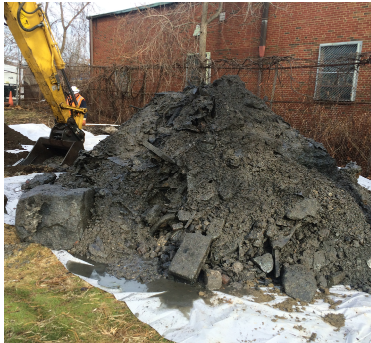
-Stockpile of waste fill material after completion of excavation.
