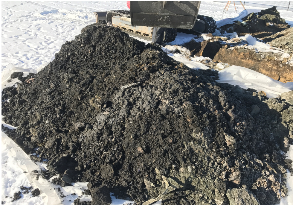
-Stockpile of waste fill material after completion of excavation.
