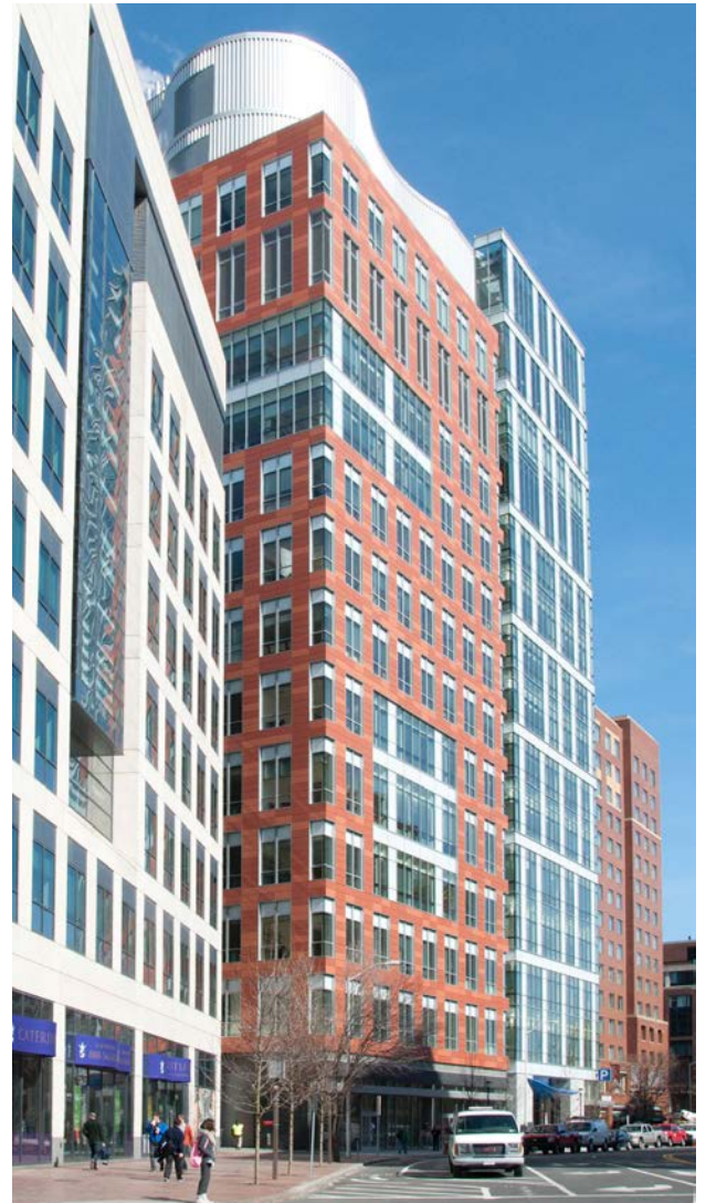
Differentiation of tall buildings into distinct elements and vertically grained facades help reduce their sense of bulk.
