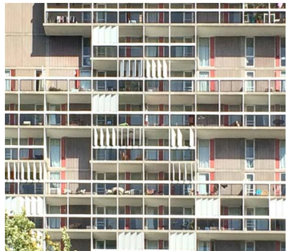
Balconies and sun shading devices can add visual interest.
