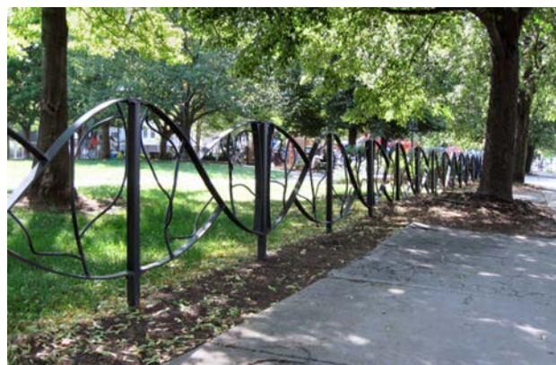
Fences enhance parks by demarcating their perimeters while offering visual connections from the bordering streets.
