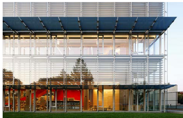
The civic role of institutional buildings may be symbolized by their iconic facades. In this example, a double glazed facade with adjustable shading mechanisms combines energy efficiency with visual openness.
