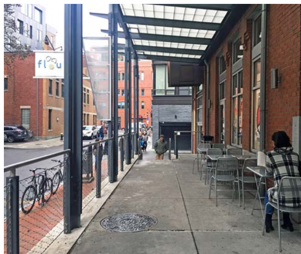
Where elevated sidewalks are provided, they should be wide and continuous to take precedence over ground level sidewalks.
