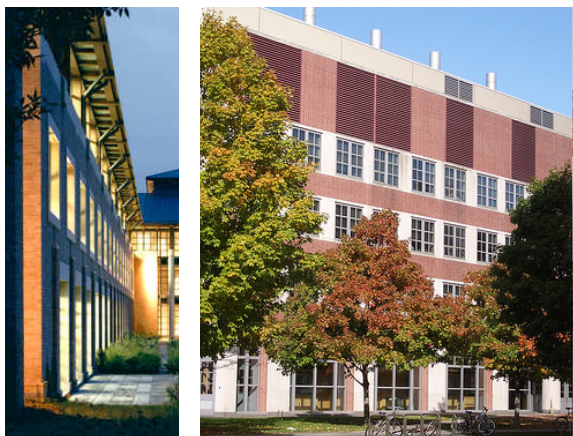
Top floors and penthouses may be differentiated to accommodate mechanical equipment or to create an expressive building top.
