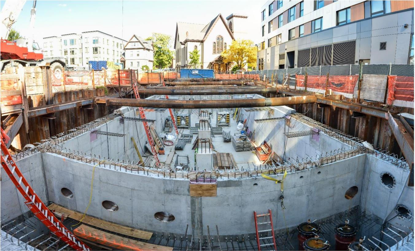
Construction on an underground tank in The Port that captured almost 3.5 million gallons of stormwater water during summer 2021
