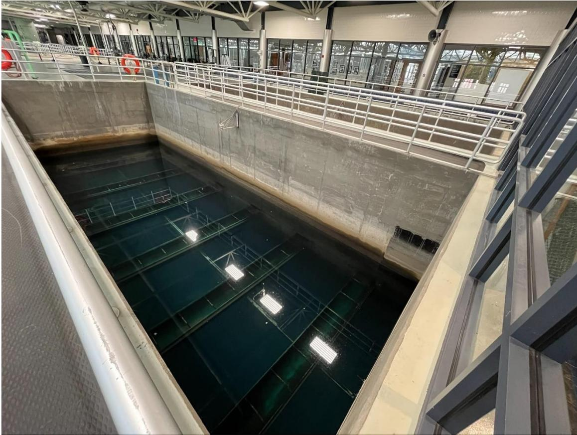
One of the water filters with newly replaced granular activated carbon media
