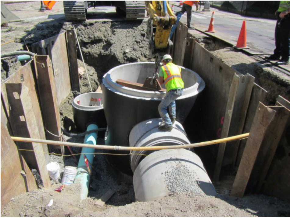
Figure C.11. Combined sewer separation in Cambridge. (Source: Kleinfelder)
