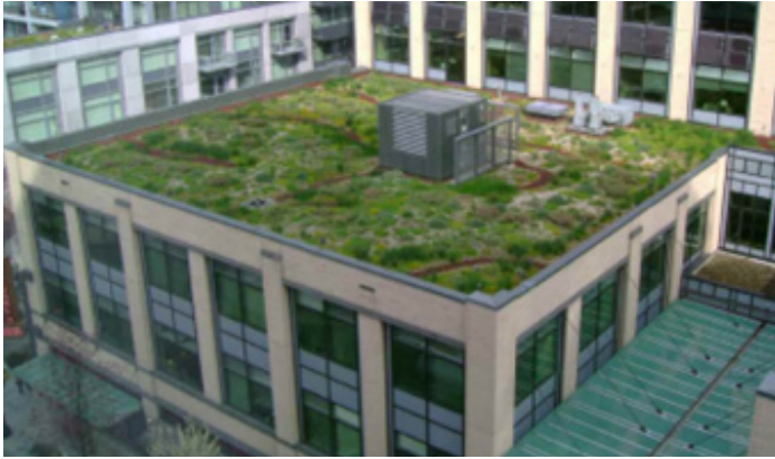
Figure C.1. Portland Green Roof. (Source: Portland Environmental Services, Portland, Oregon)
