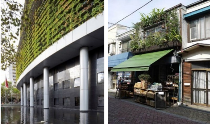
Figure D.3. Green wall on a building in Concepción, Chile, (left) and a green wall on a small business building on Shin-Koenji street in Tokyo, Japan (right). (Sources: inhabitat.com/consorcio-headquarters-by/ ; tokyogreenspace.wordpress.com/ )
