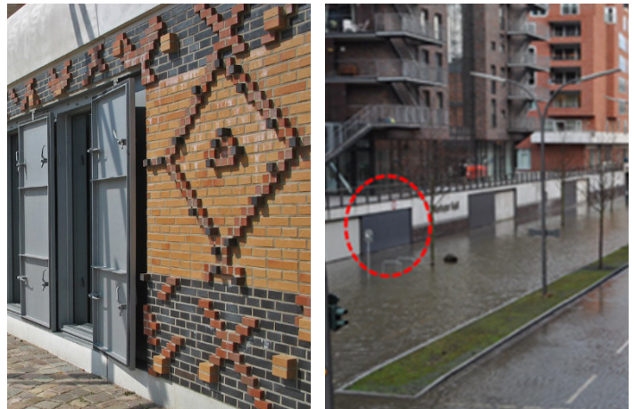
Figure B.2. Flood protection shutters. (Source: HafenCity, Hamburg)
