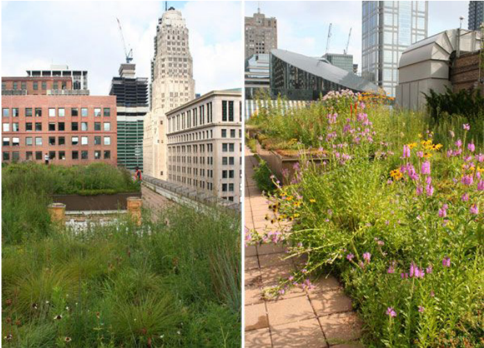
Figure D.4. Chicago Green Roof. (Photo credit: Conservation Design Forum)
