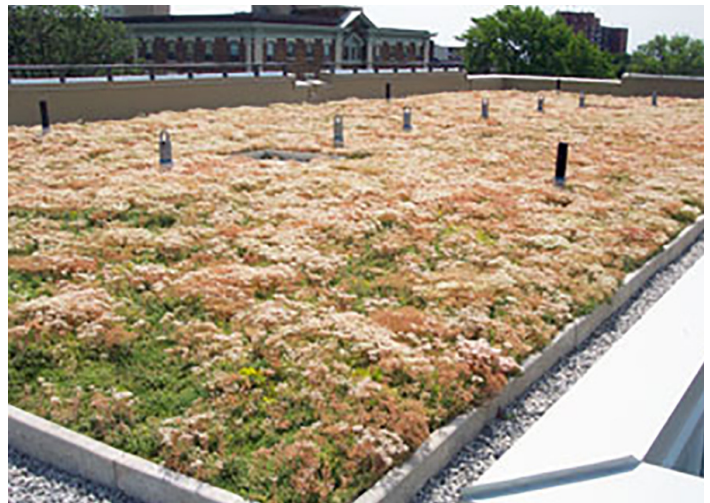
Figure B.6. Green roof system. (Source: Toronto, Canada; Green Roof at Ryerson University)
