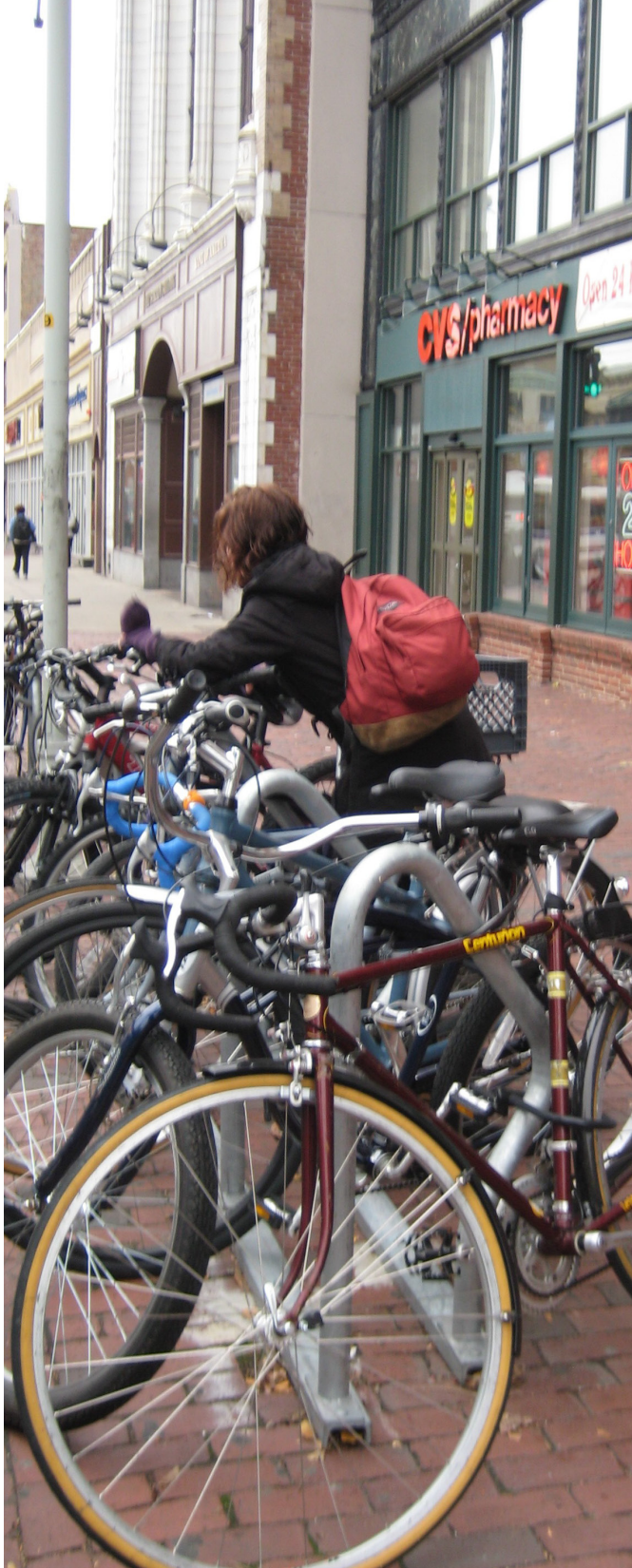
Figure 7.2: The “Swerve” rack on a rail system enables racks to be located where it is not feasible to drill into pavement.
