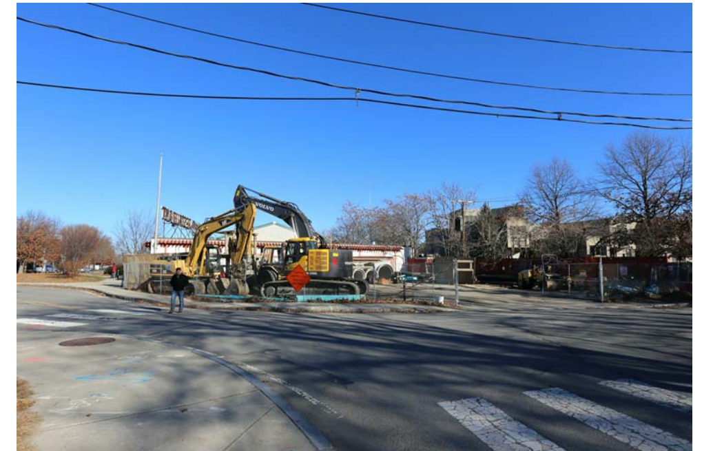
VIEW TOWARDS SITE FROM VASSAL STREET
