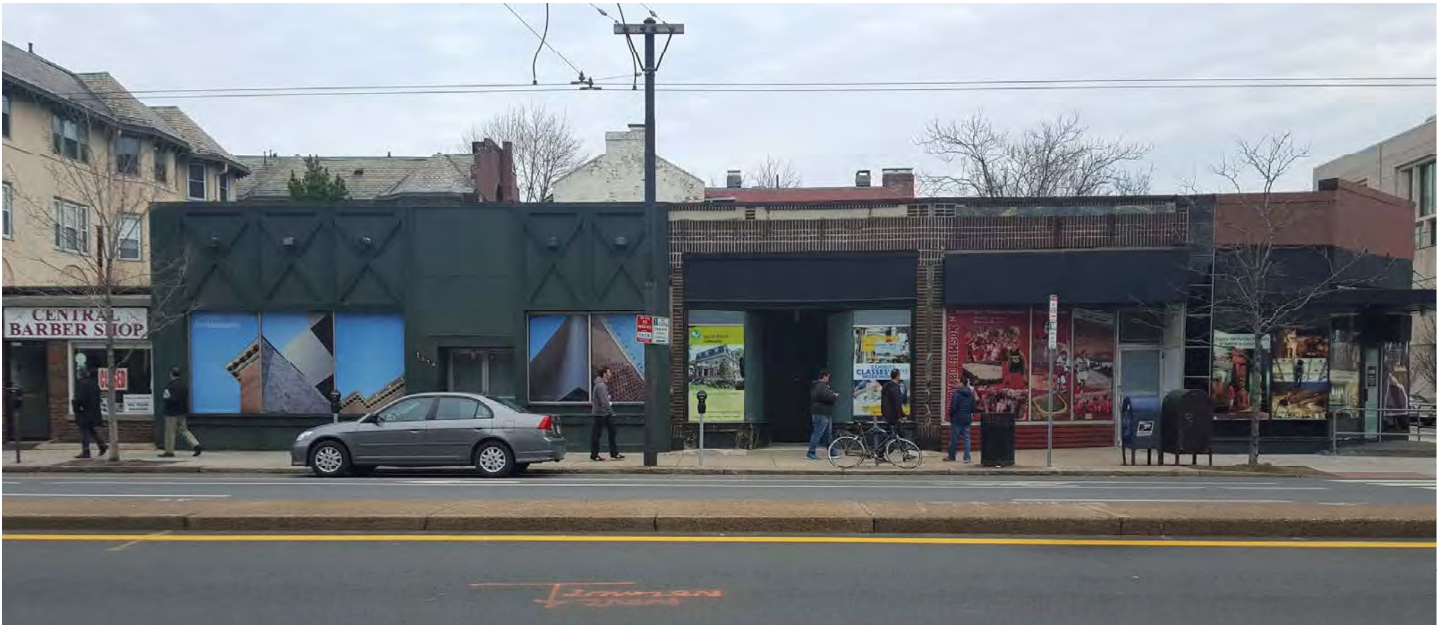
05 View across Mass. Ave. of existing 1607-1615
