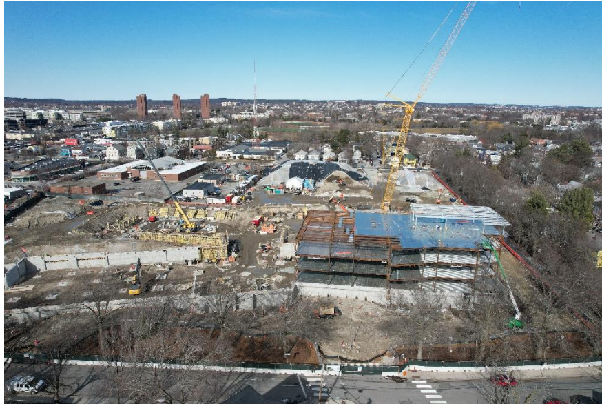
The Tobin Montessori & Vassal Lane School, under construction
