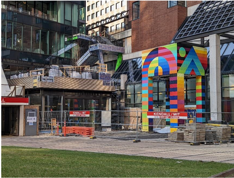
Ongoing work at the Kendall Square MBTA Station
