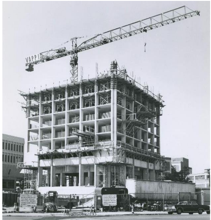
Eastgate during construction, August 1966. Image courtesy of MIT Museum.
