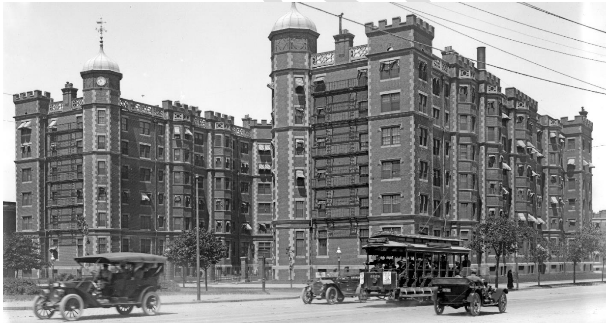
Riverbank Court Hotel
