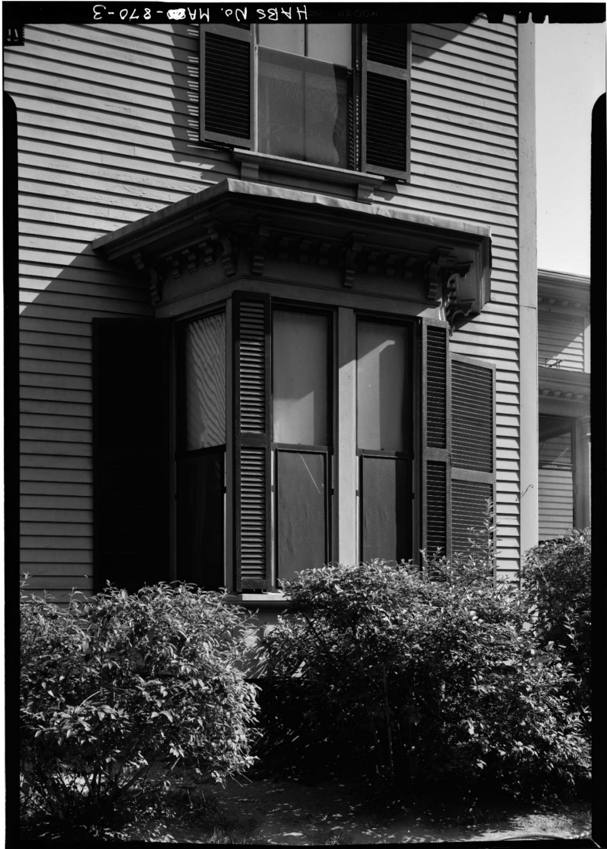
Detail of bay window. HABS photo, 1964.
