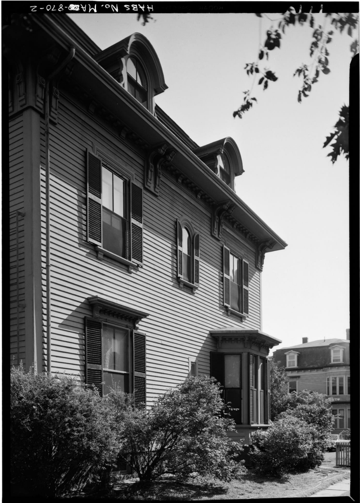
South elevation, from the southeast. HABS photo, 1964.
