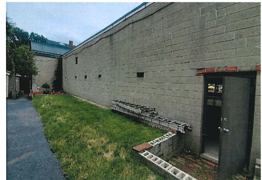
REAR ELEVATION EXISTING CONDITIONS- THIRD BUILDING
