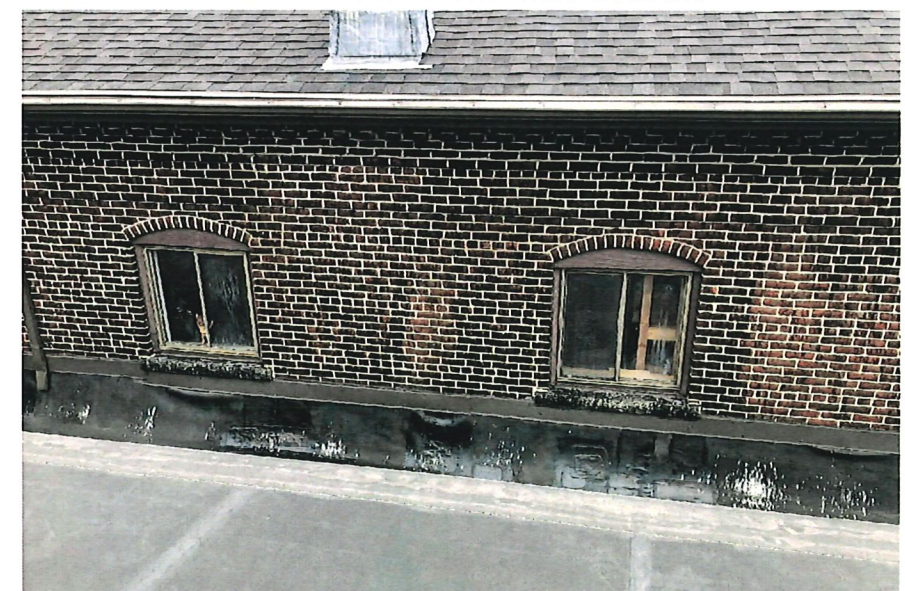
BARN LEFT SIDE - WINDOWS TO BE REPLACED
