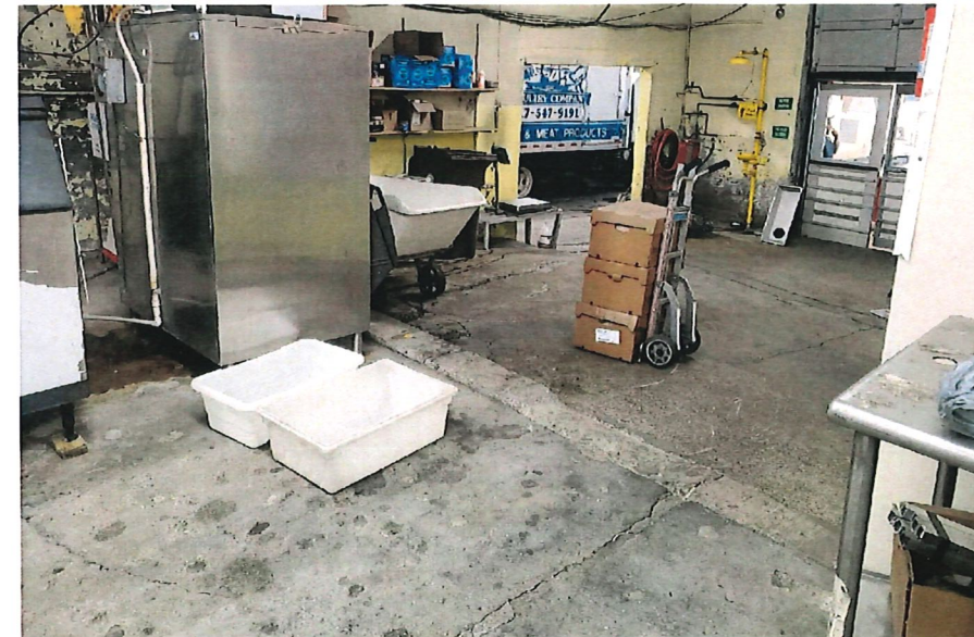
MIDDLE BUILDING EXISTING FLOOR SLABS
