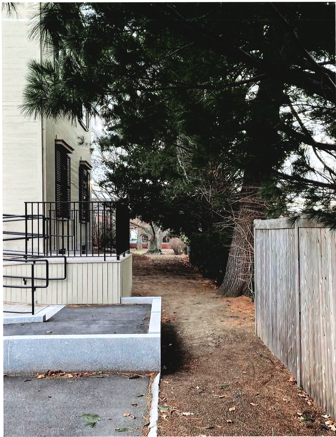
EXISTING CONDITION | VIEW OF 101 BRATTLE SIDE YARD
