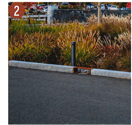
BITUMINOUS CONCRETE PAVING
