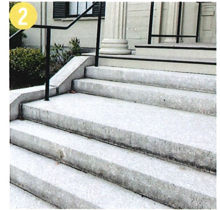
REPAIRED OR REPLACED GRANITE STAIRS
