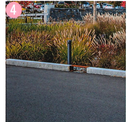
BITUMINOUS CONCRETE PAVING
