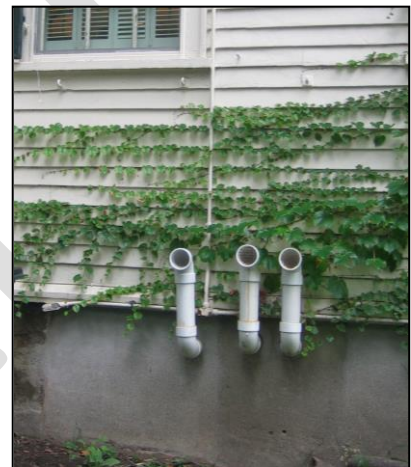
Figure 4: Highly visible PVC vent pipes
