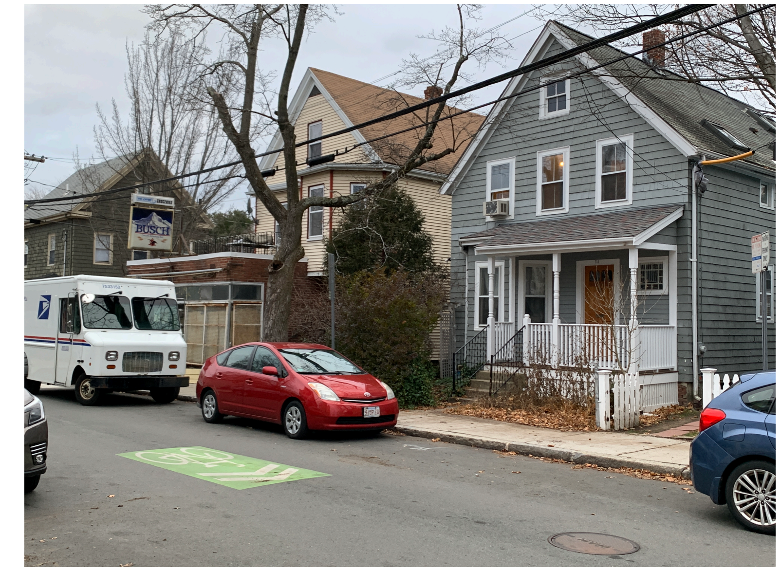
View Towards Site Via Dudley Street
