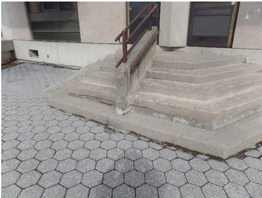
Photo 18: Unit C South Entry Stair
