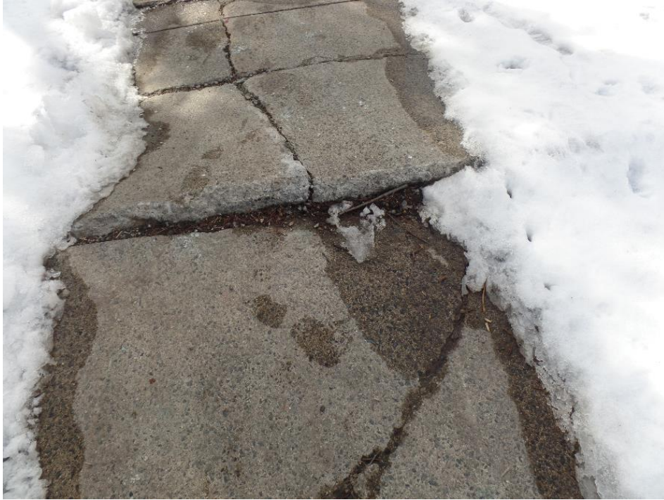
Photo 19: Cracked/Frost-Heaved Sidewalk
