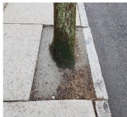
TREE PLANTED TOO LOW AND INADEQUATE SOIL VOLUME
