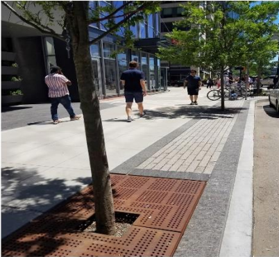
BOYLSTON STREET, BOSTON TREE PLANTING ZONE WITH PERMEABLE PAVERS AND TREE GRATES
