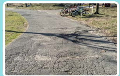
Repave all paths and resurface pavement
