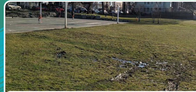
Address the persistent drainage issues in the field
