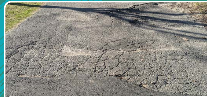
Repave all paths and resurface pavement
