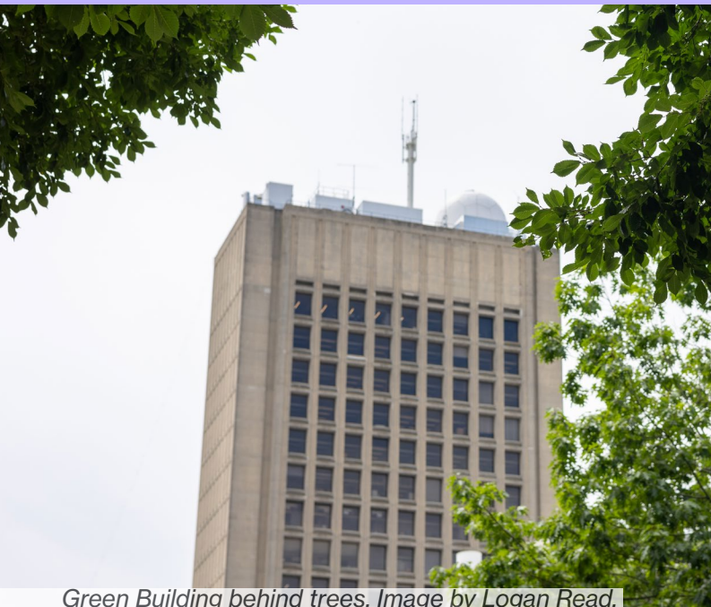
Green Building behind trees. Image by Logan Read.
