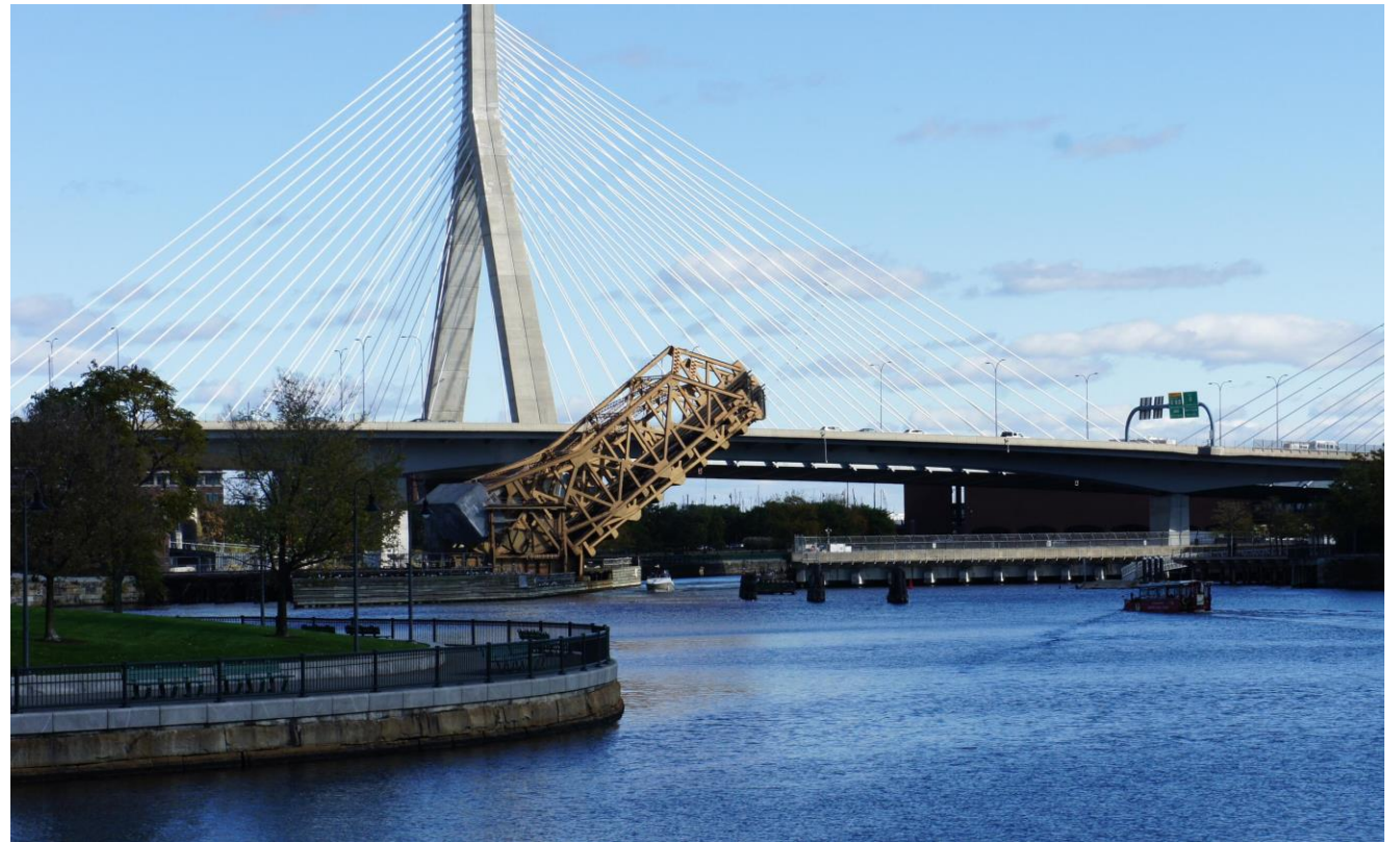
Image: MBTA Draw One bridge on the lower Charles River Basin Source: MBTA
