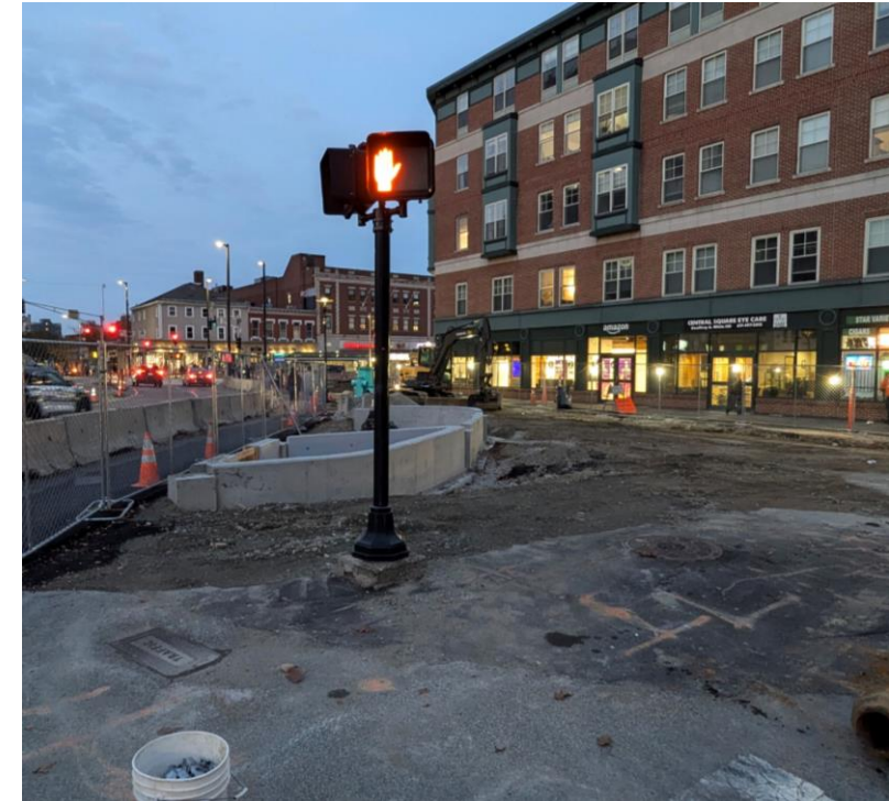
Bus Terminal construction work zone where there were previously boarding islands
